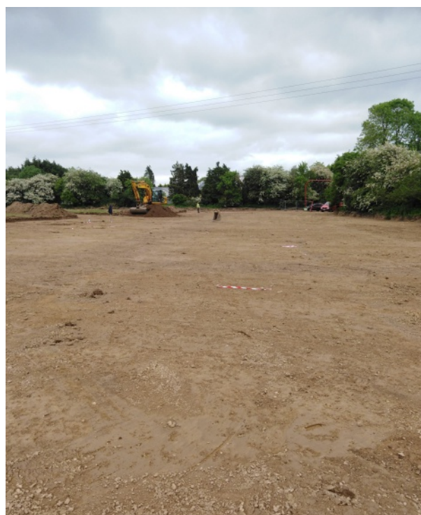
Monitoring in Field 2, looking east
