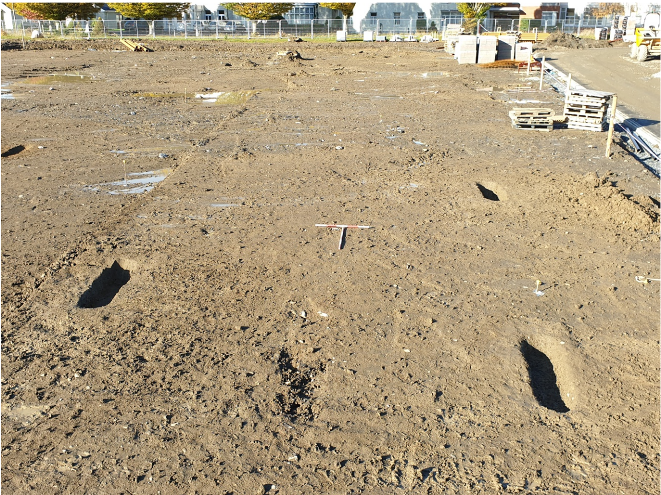
Area 6 overview facing northwest
