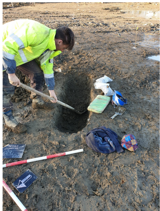
One of the Clonsilla pits under excavation
