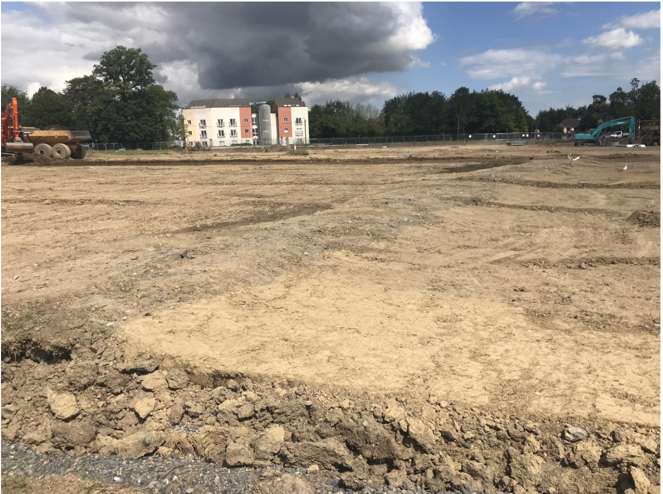
View of general monitoring programme, showing removal of topsoil down to natural subsoil
