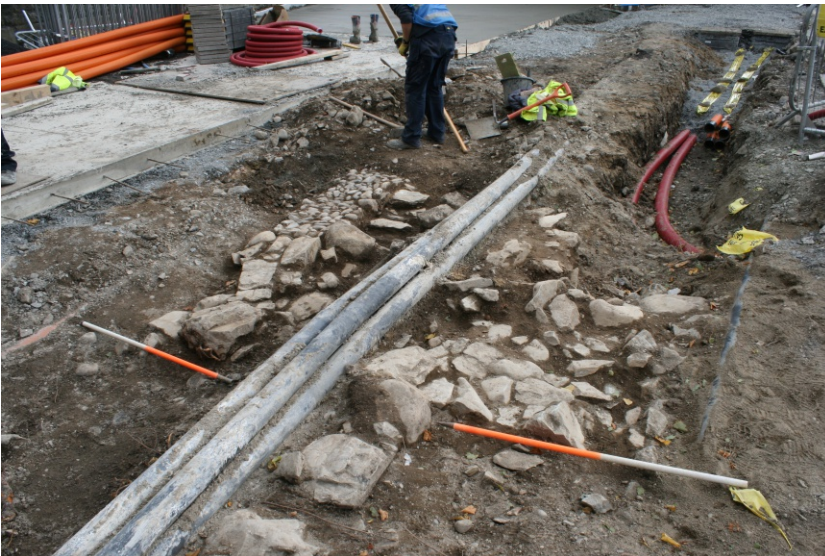
Church of Ireland facing south, showing medieval towerhouse wall C140
