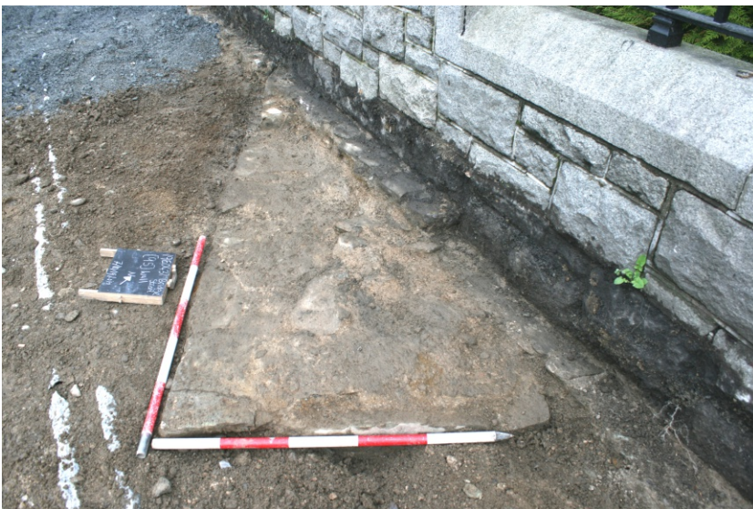
Bridge Street wall C95
