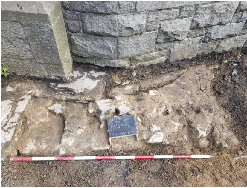
Bridge Street wall C83
