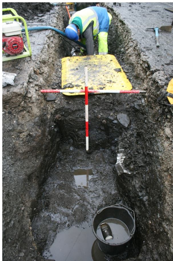
Church Street working shot
