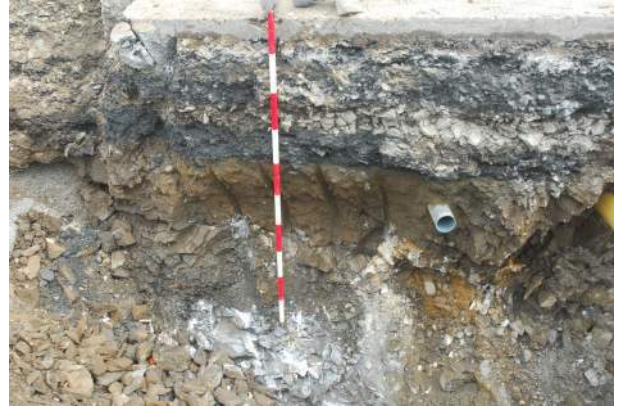
Working shot of service trench excavated across Drumree Road, with ditch C503 surviving in section below road gravels, truncated by a water pipe to the right (top)
