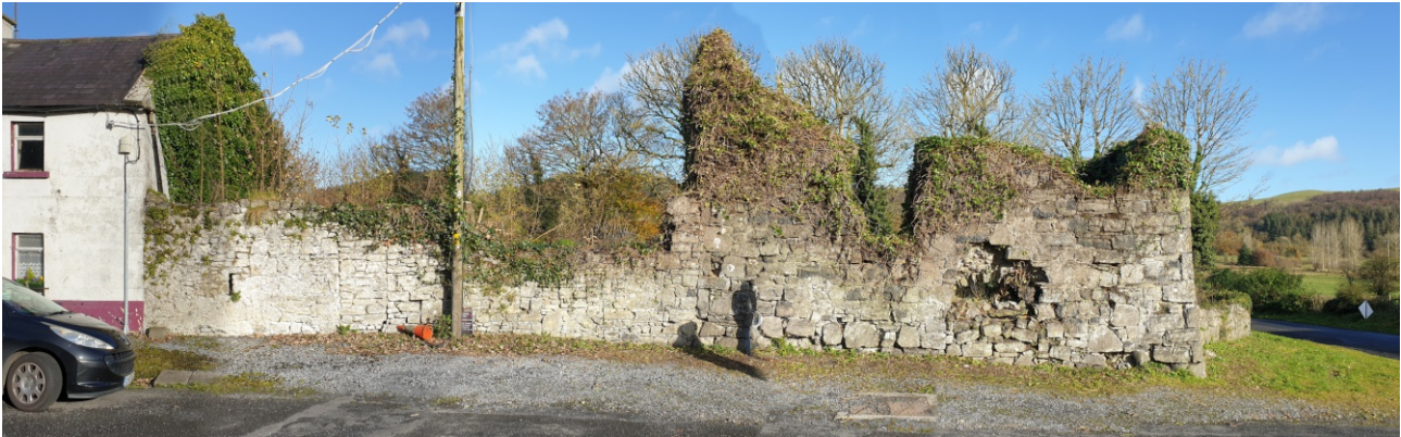
Combined photograph showing front facade (south-facing) of Fore Gaol
