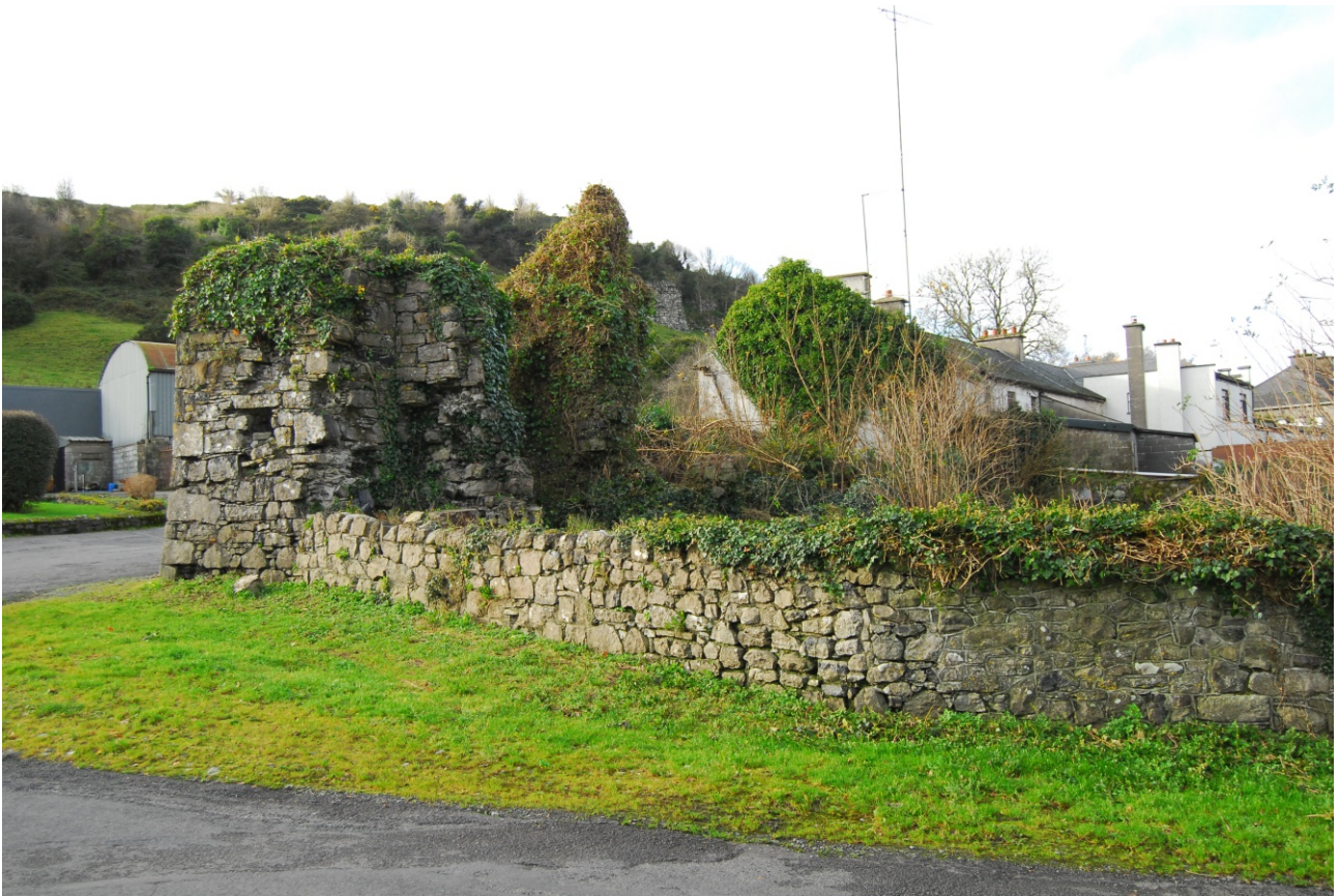
View of eastern end of building, showing later roadside wall
