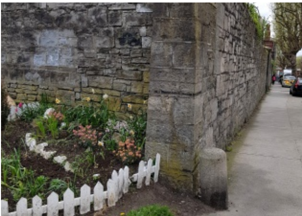
Northwest corner with gate pier and bollard
