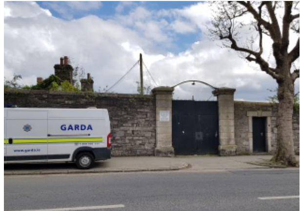
Southern gate on western boundary wall
