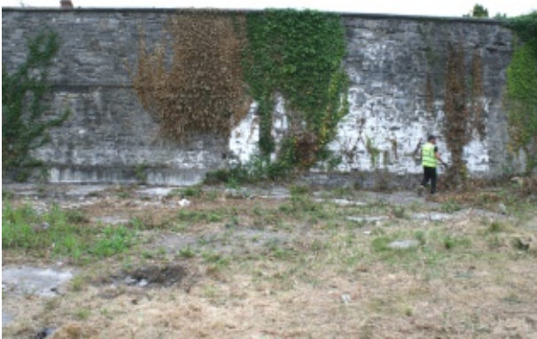
East boundary wall interior
