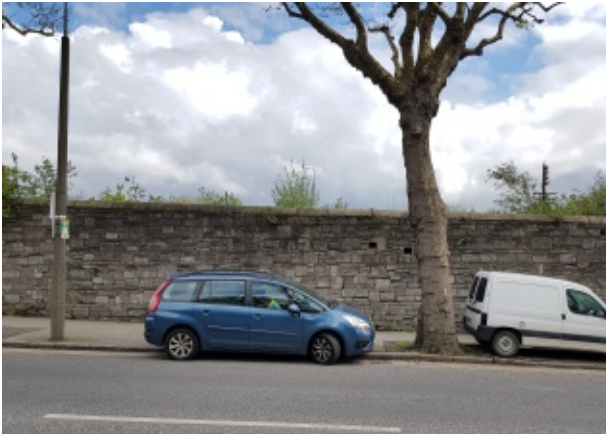
West boundary wall exterior
