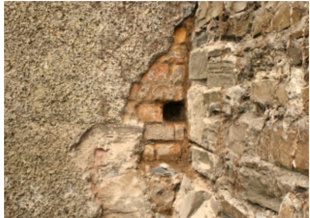
Militia Barracks, yellow brick blocking former coal cellar
