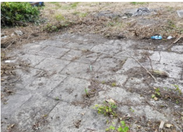
Granite paved floor of Engine House
