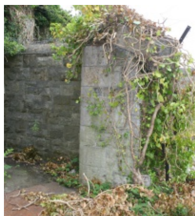
Masonry corner of stores adjacent to Married Quarters
