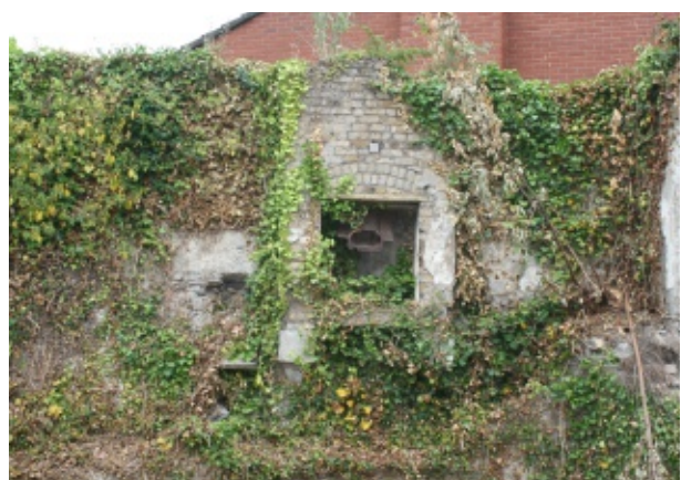
Remains of Control Office fireplaces in east boundary
