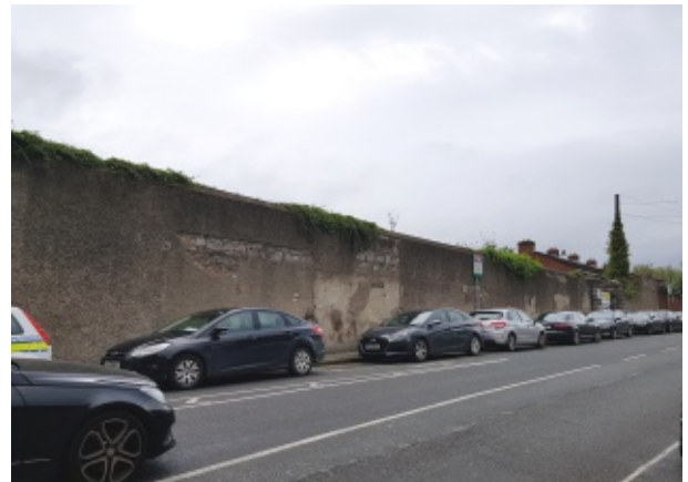
Southern boundary wall exterior
