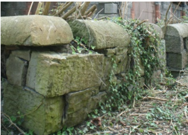
Retaining wall adjacent to Married Quarters
