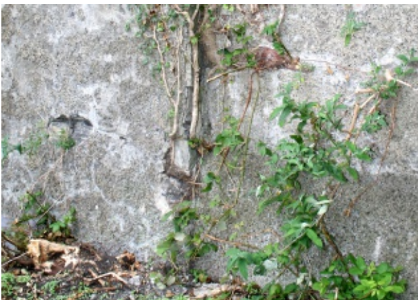
Militia Barracks, scar of former wall and early brick
