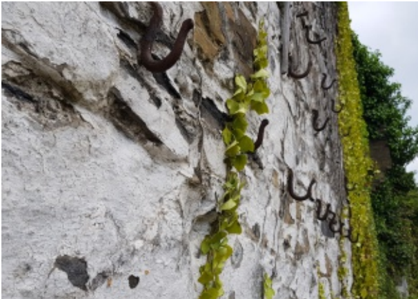
Hooks from Engine House on east boundary
