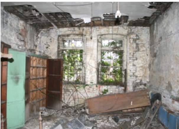
Militia Barracks, interior of earlier eastern section
