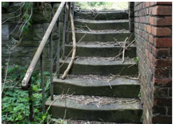
Granite steps adjacent to Married Quarters
