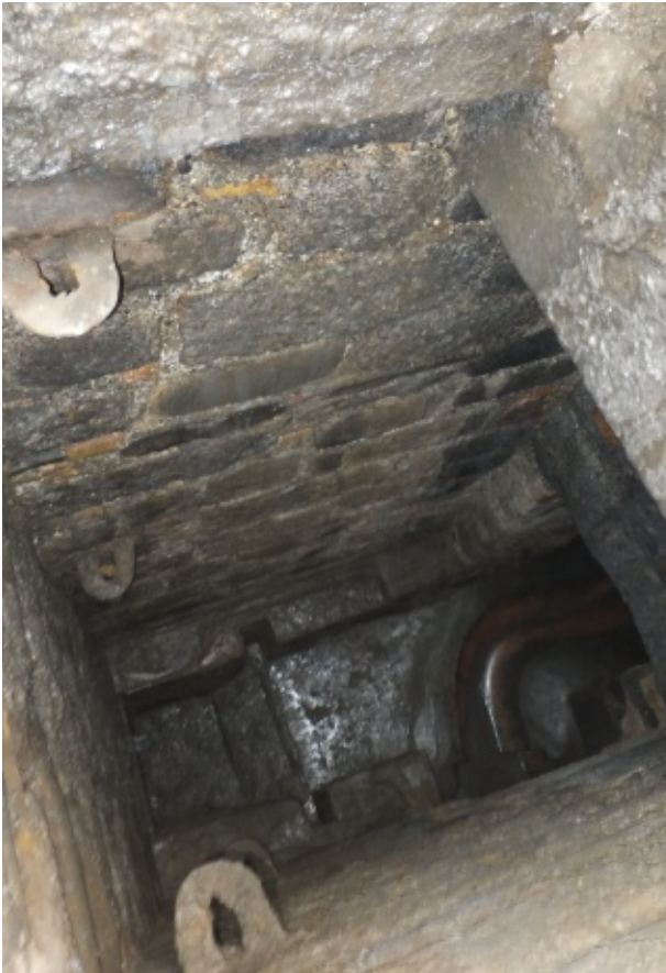
view into deep water culvert running east-west under James' Gate
