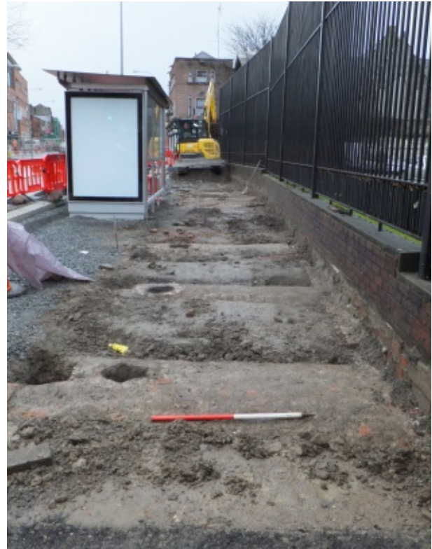
cellar crowns at Nos. 115-116 James' Street
