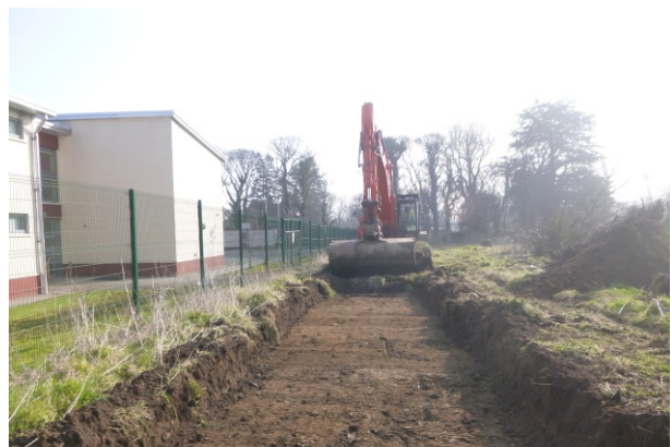
Field drain within northern trench, looking north (top)
