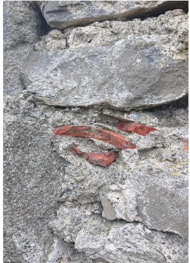
C18th coarse white lime mortar in the original gate pillars
