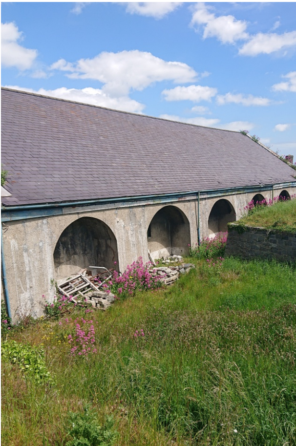
Pallets south of Magazine Store Building A
