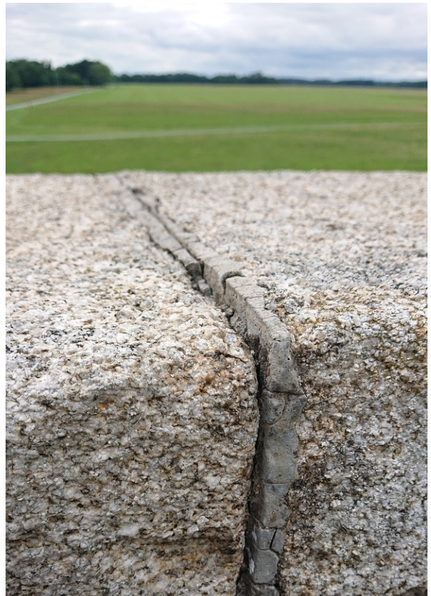
C20th Blue cementitious mortar used in rampart repairs
