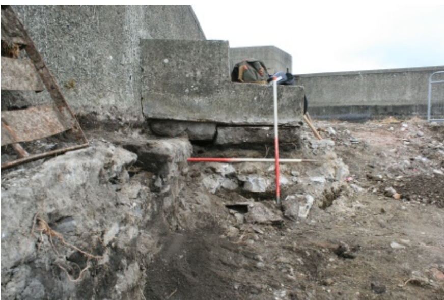
Profile below concrete walkway, showing gun platform and masonry fill directly below concrete
