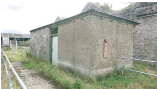
Building G exterior
