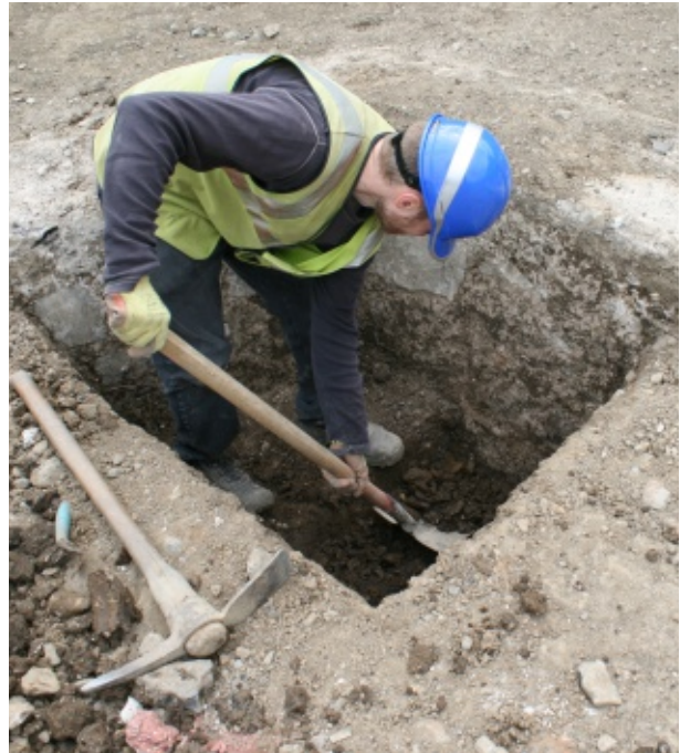
1m by 1m hand-excavated square test-pit through later rampart fill (C9)
