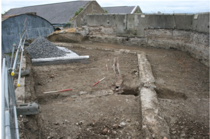
Overview of gun emplacement drainage, facing south
