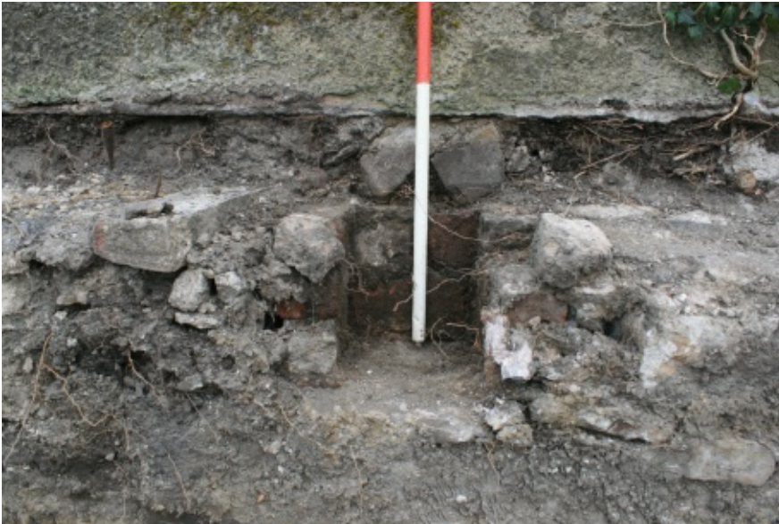
Gun emplacement drain base cut into outer rampart wall
