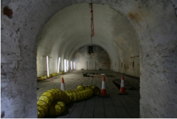
Magazines Store A facing west
