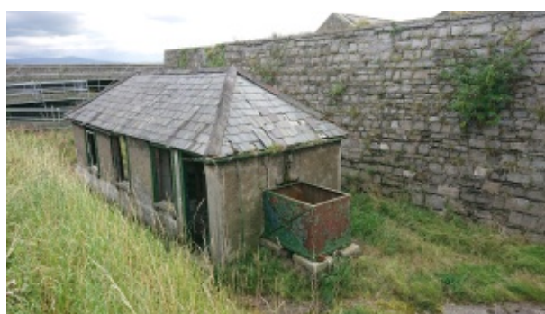
Building F exterior showing water tank, possibly replacing 19th century cistern
