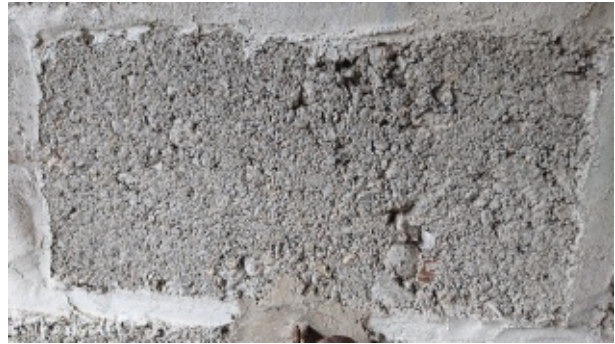
The concrete blocks used for the Paxo Plant walls in Building B have high levels of large inclusions, which may relate to the shortage of coal and raw materials at the Drogheda concrete plant
