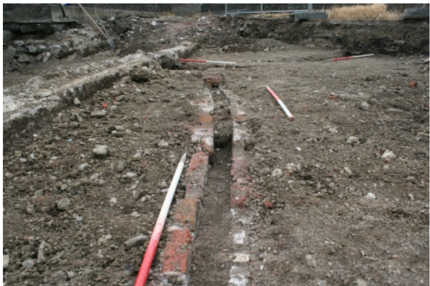
Detail of brick-lined part of drain
