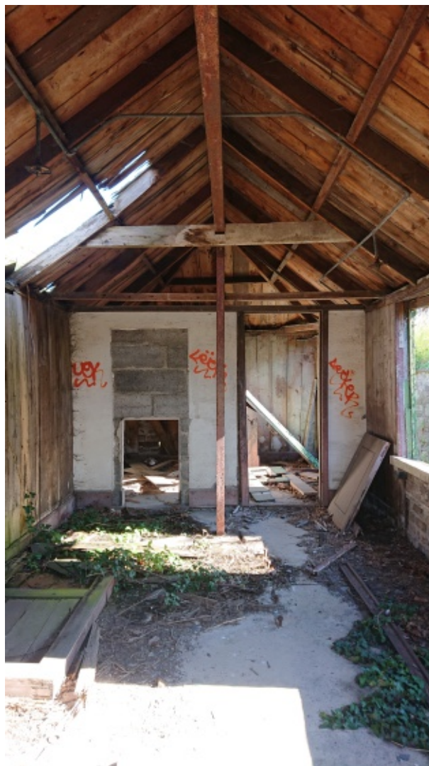
Building F interior showing steel frame, possibly c. 1940s
