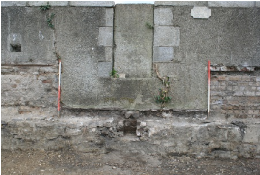
Detail of gun emplacement following ground reduction
