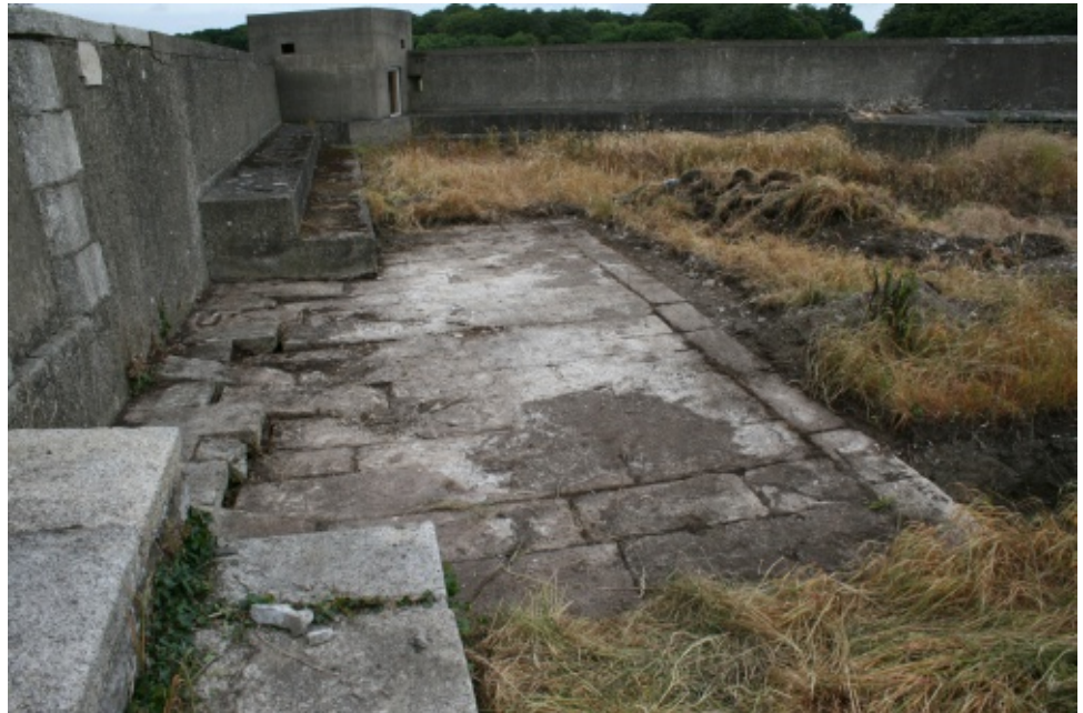
Area C gun platform CC2 prior to lifting
