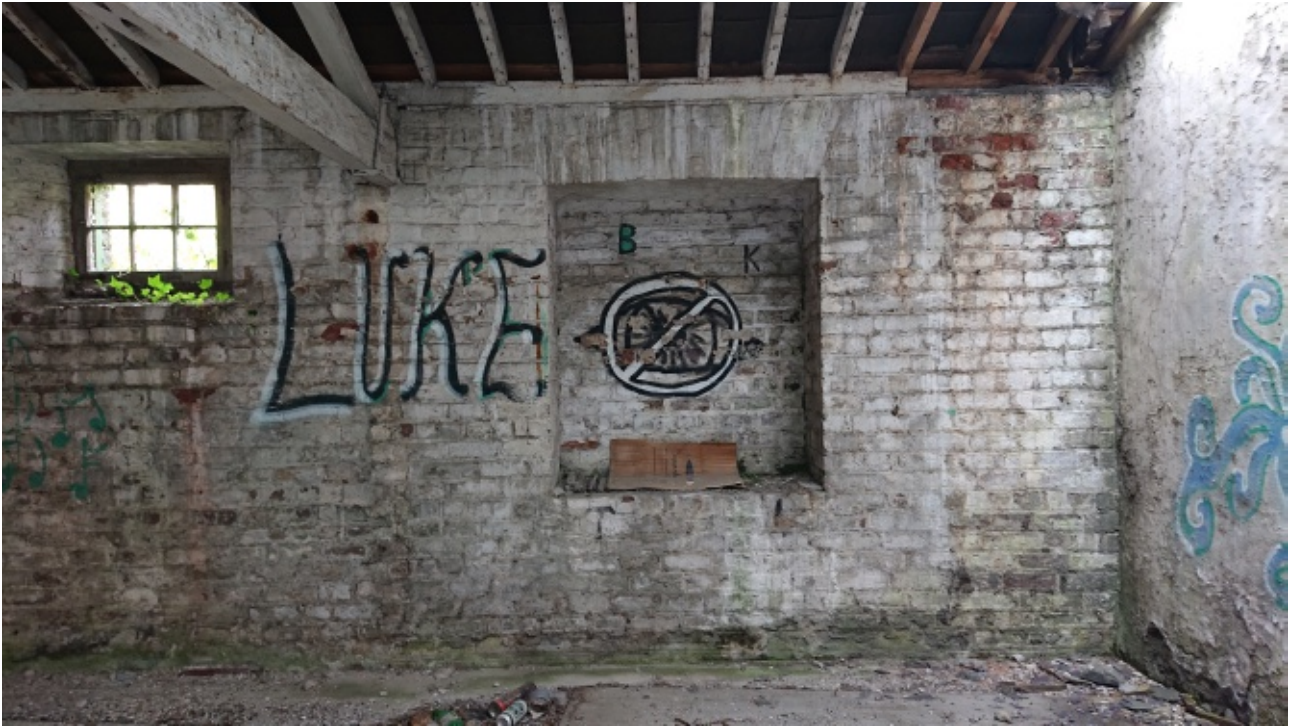
Building C, western side, showing remains of wooden partition of fireworks c. 1901 store to left of image, removed in the 1940s. Note also letters B and K in the niche.
