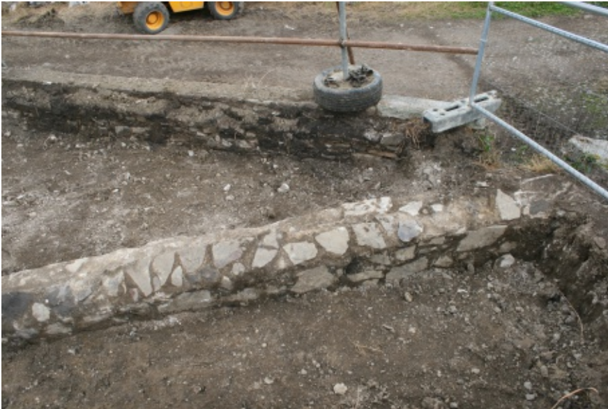
Detail of early (1736) rampart retaining wall
