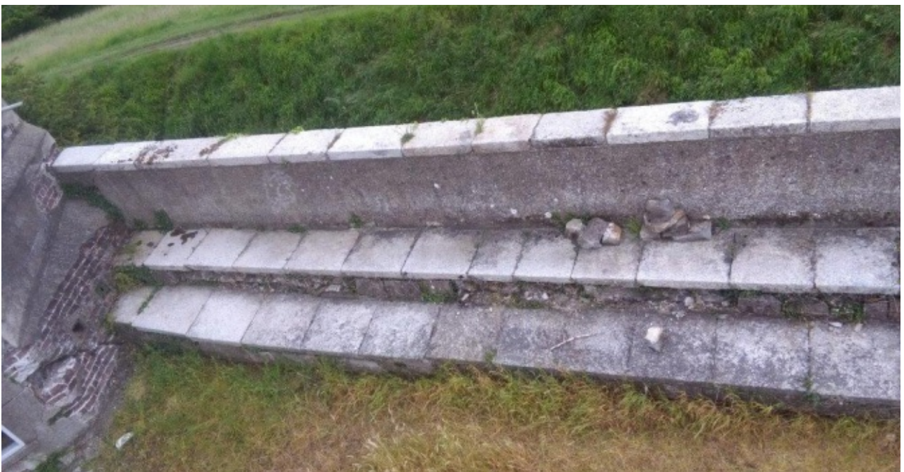
Area A walkway prior to lifting
