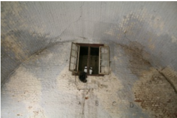
Rear window of Building A, frame C11 comes from here
