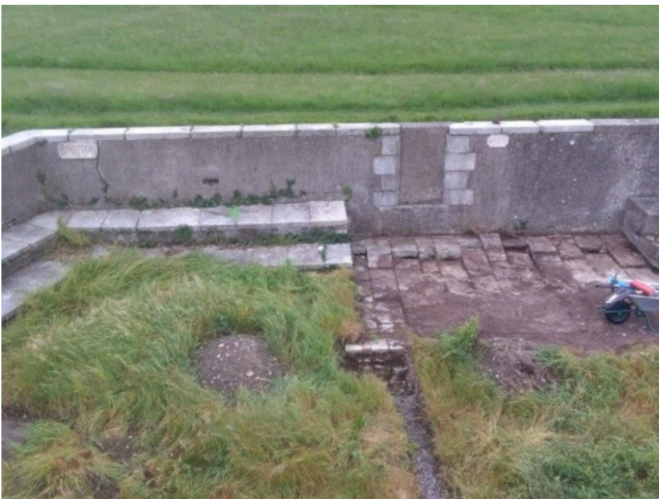
Area C walkways and platforms prior to lifting
