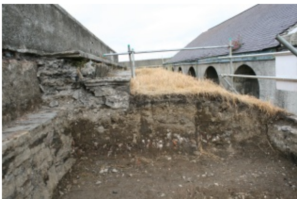
Rampart ground reduction in Area A
