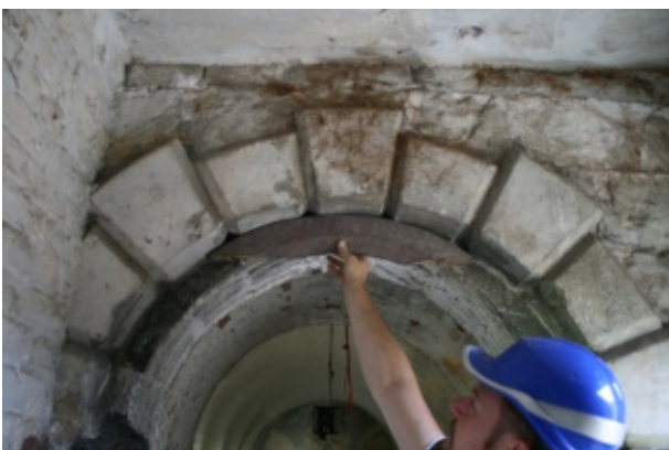
Front door Store A, frame C12 comes from here
