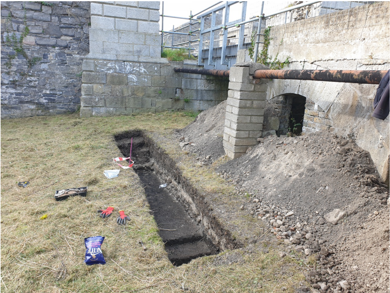
Overview of test-trench 3, facing northwest
