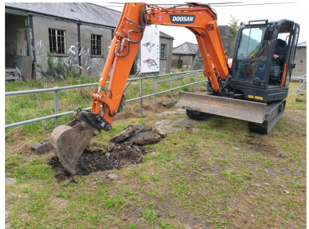
Excavation of concrete test pit 1
