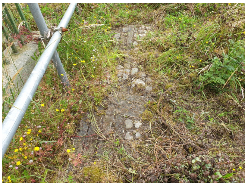
19th century brick gutter outside building K
