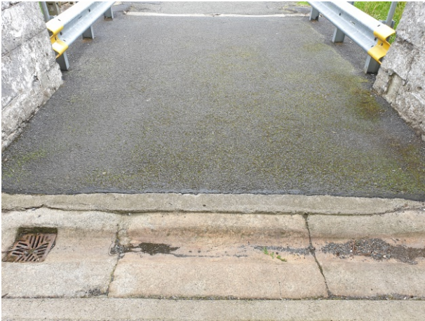
Granite gutter at entrance to ravelin
