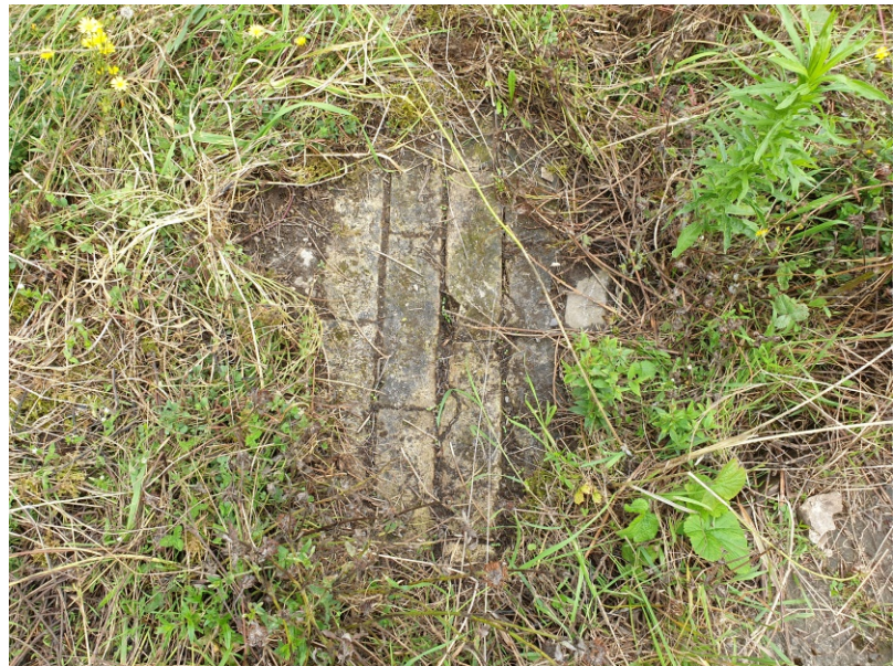
20th century brick gutter repair outside building K
