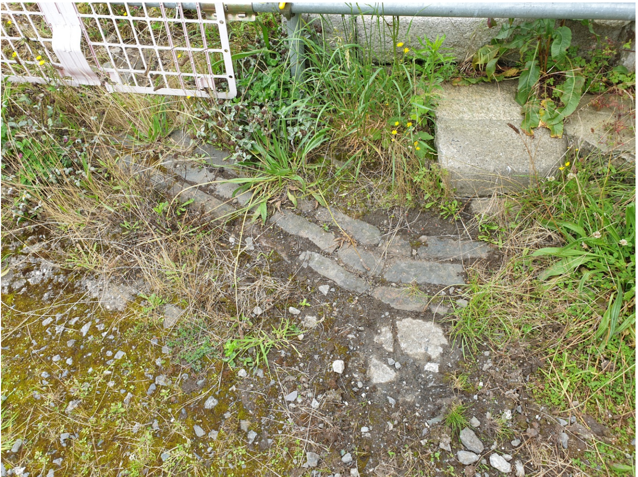
Stone setts lining gutter at entrance to ravelin
