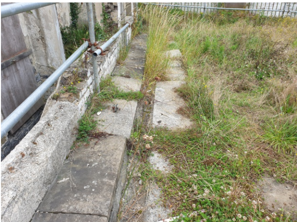
Granite gutter outside building K
