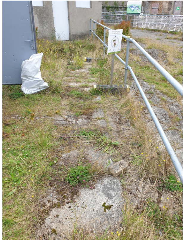
Granite 'sentry walk' to south of concrete driveway in ravelin
