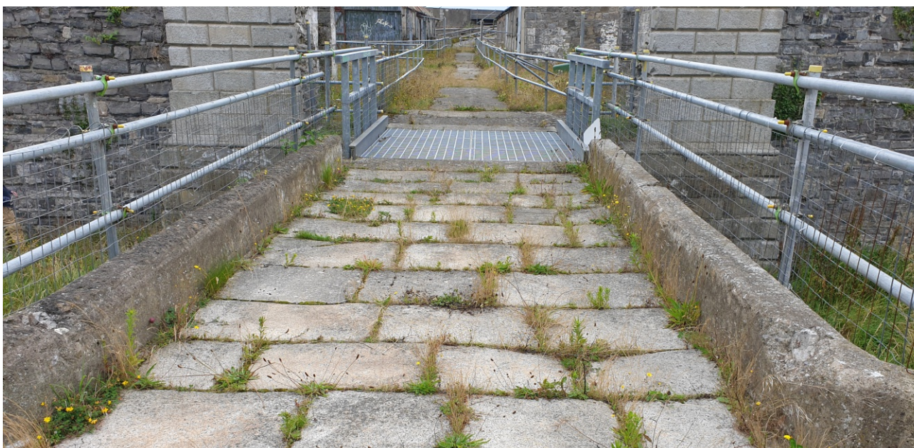
Granite pavement over bridge from ravelin to main fort
