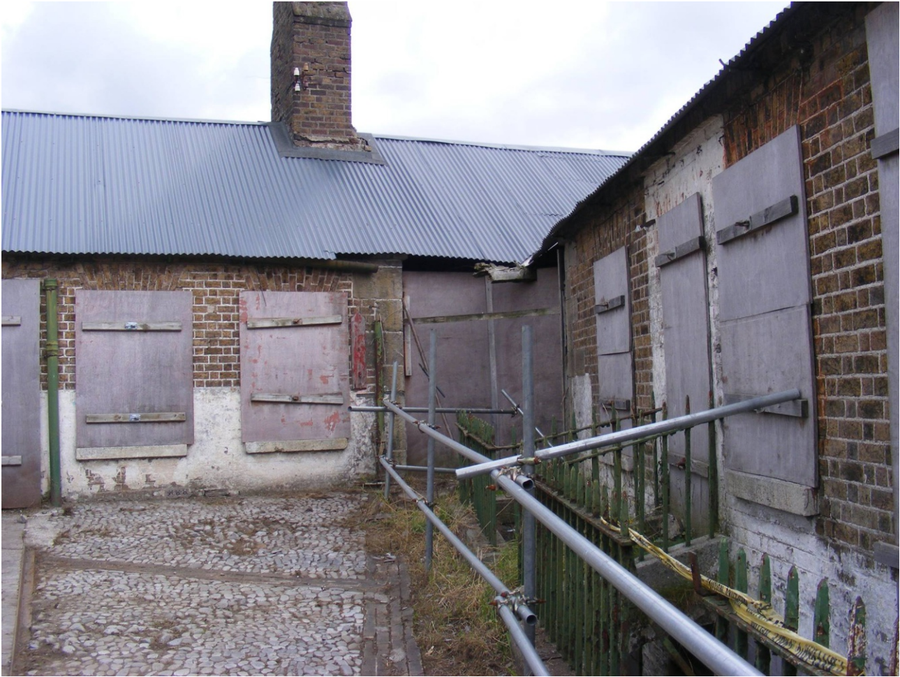
Cobbles in ravelin, from Noel Fitzgerald 2017 ('save the magazine fort' facebook page). Note brick-lined gutters, in contrast to cover image which shows possible cobblestone gutters in lower left and lower right.
