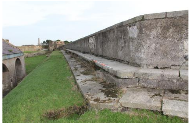
Looking E along rampart platform at E end of Area B.
