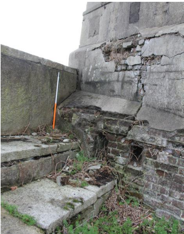
Junction of rampart platform and SW cavalier.
