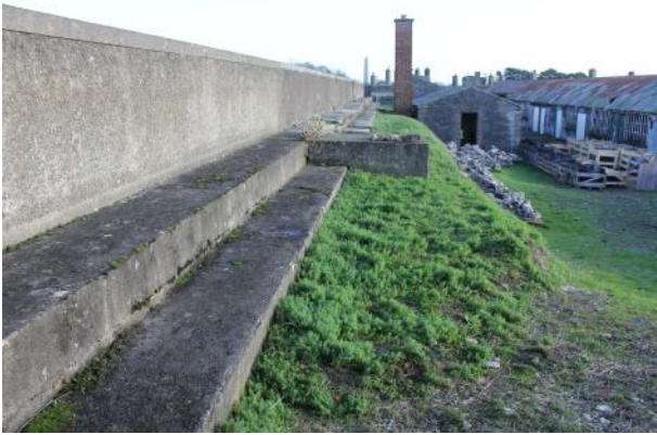
View E along S-facing rampart walkway.
