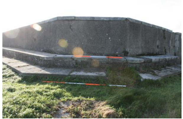
NE-facing segment of parapet walkway.
