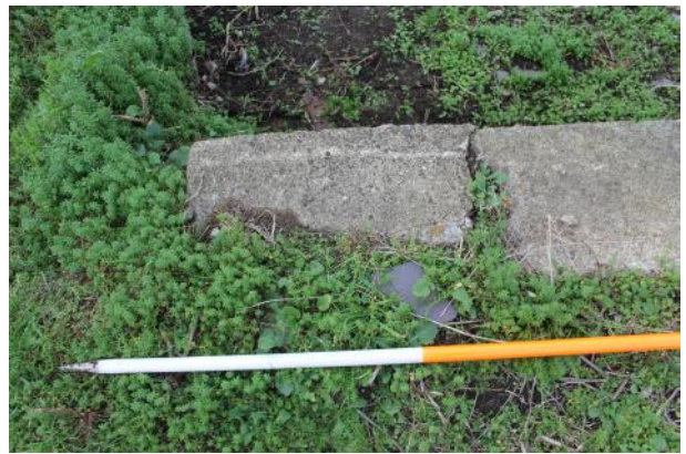
Detail of concrete capstone at S end of W-facing wall.
