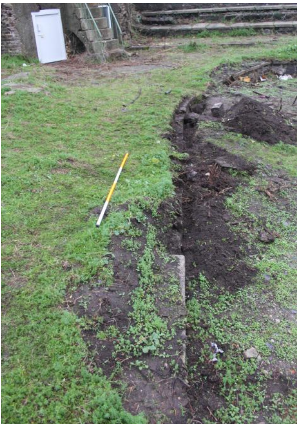
Trench 4 looking W.
