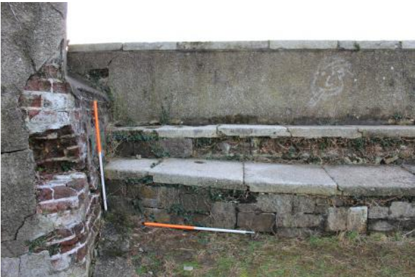
SE cavalier showing junction with walkway.
