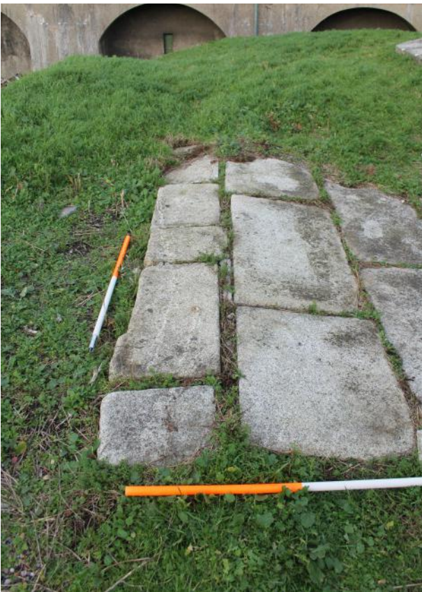
Detail of W end of gun emplacement platform. Note shorter slabs at W end of platform.
