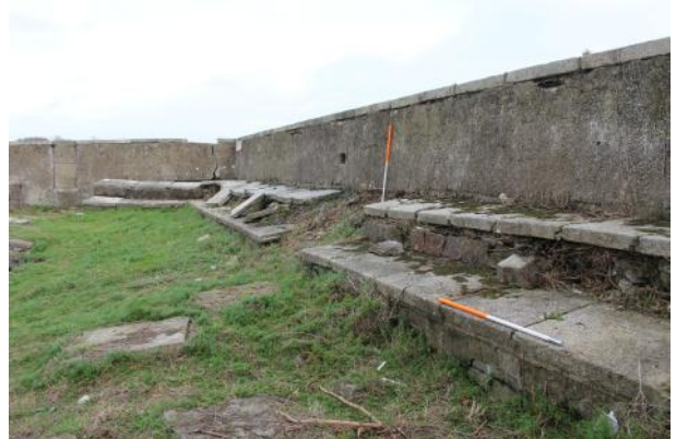
Looking E along the S wall of the SW bastion.
