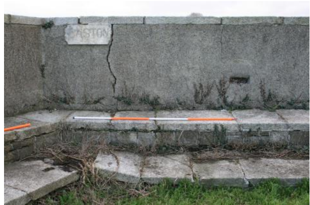
NE-facing segment of parapet walkway.
