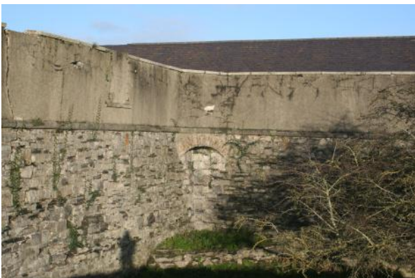
Area B, junction of SW cavalier with S wall of fort. Note squinch and gun embrasure.
