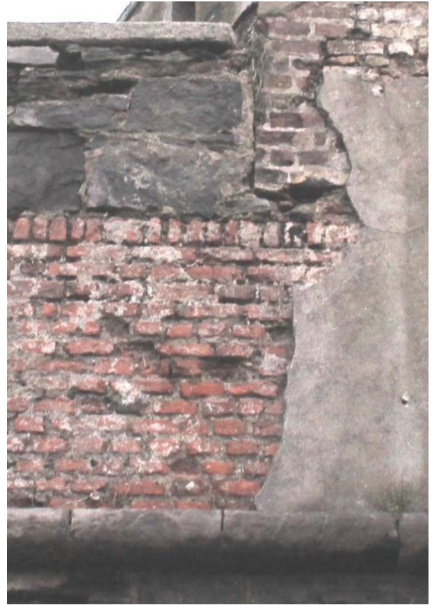
Area A, external view of SE cavalier looking SW, detail showing masonry over brick in parapet
