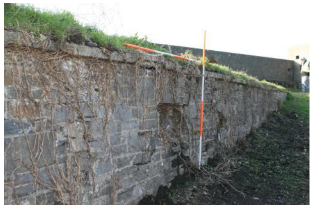
View along NE-facing rampart retaining wall.
