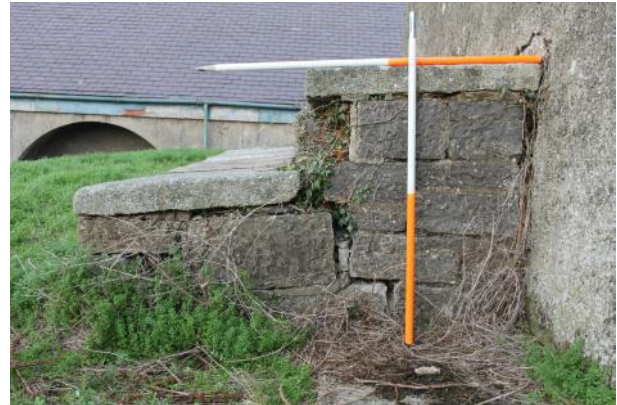
Terminus of rampart platform to N of gun emplacement.
