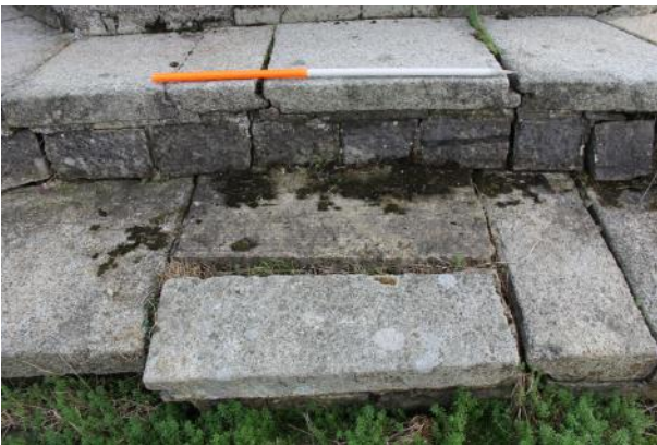
Half concrete slab inserted into lower step at NW-facing segment.
