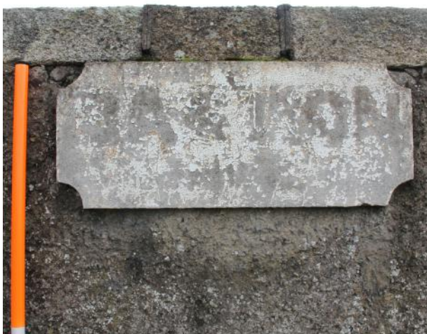
Cement BASTON sign in E end of S wall of bastion.
