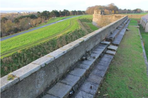
View W along the stepped rampart walkway from the SE cavalier.
