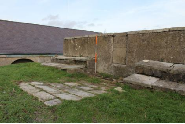
Gun emplacement in W-facing wall of bastion.
