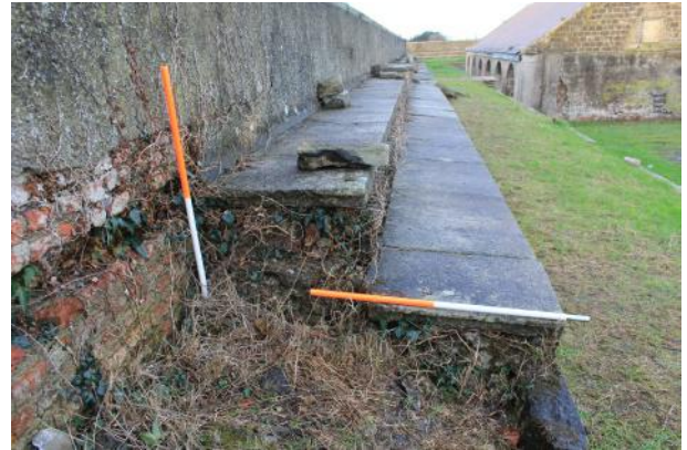
Rubble core of parapet walkway visible at breach in the feature. Looking W.
