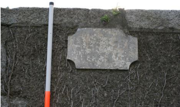
Detail of illegible cement plaque at S gun ope.
