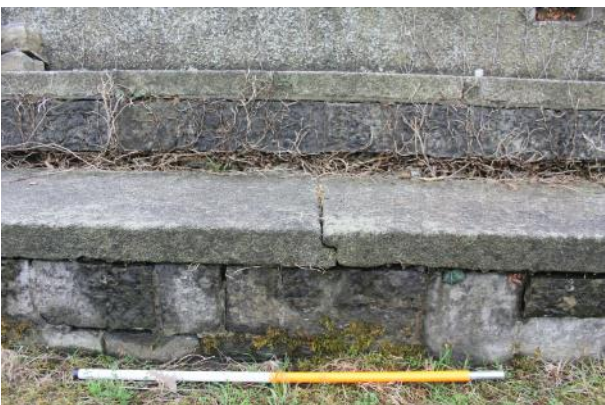
Detail of well preserved section of stepped walkway.
