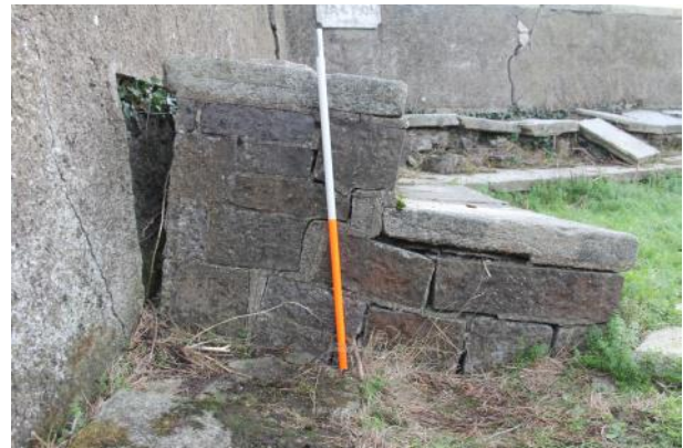
Terminus of rampart platform to S of gun emplacement. Note how the walkway has tilted forward due to subsidence.
