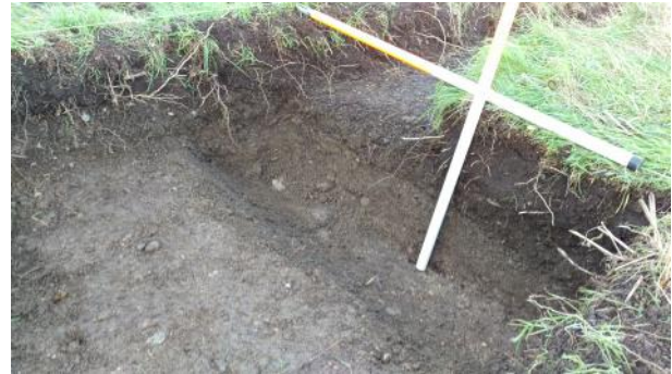
Trench 5, cut for path
