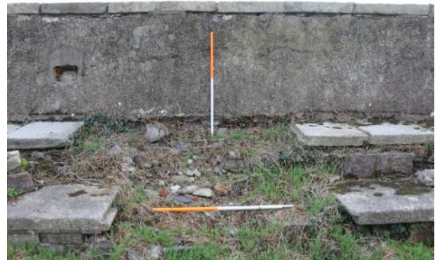
Terminus of rampart platform to S of gun emplacement. Note how the walkway has tilted forward due to subsidence.
