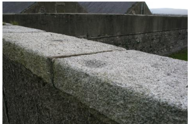
Detail of granite capstones. Note circular indentations along the internal edge of the stones.
