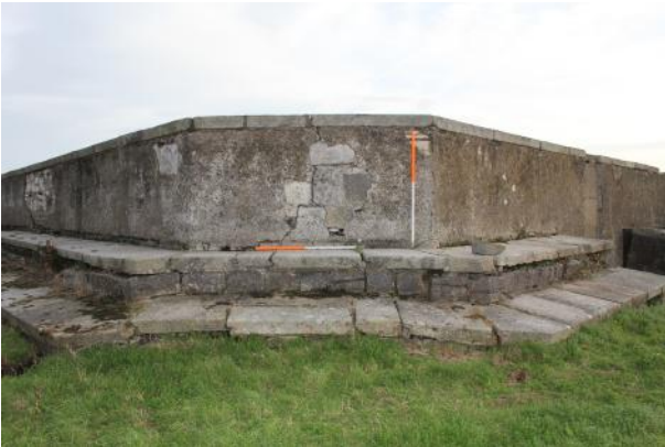
NW-facing segment of rampart walkway in Area B.
