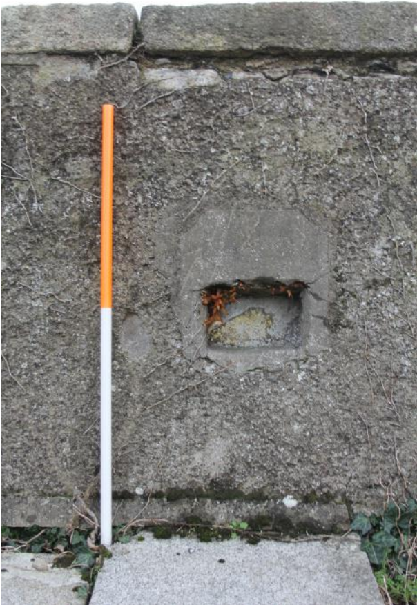
Rectangular cement-lined niche in W end of S wall of fort.
