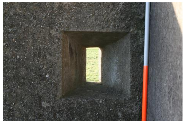
Detail of gunloop in parapet wall immediately SE of NW cavalier.
