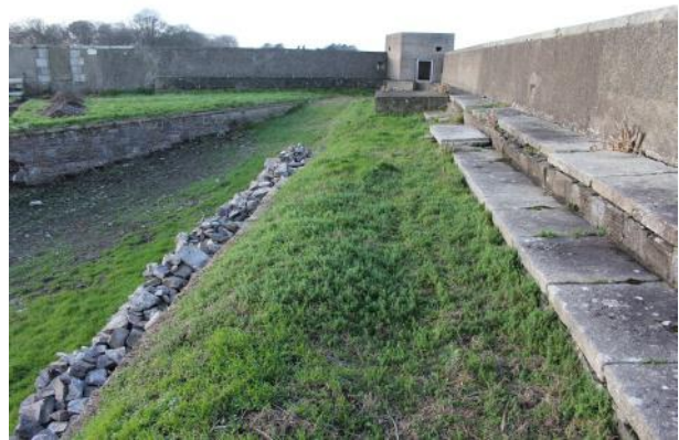
Rampart platform of S-facing wall. Looking W.
