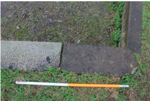
Concrete capstone at E end of rampart retaining wall.
