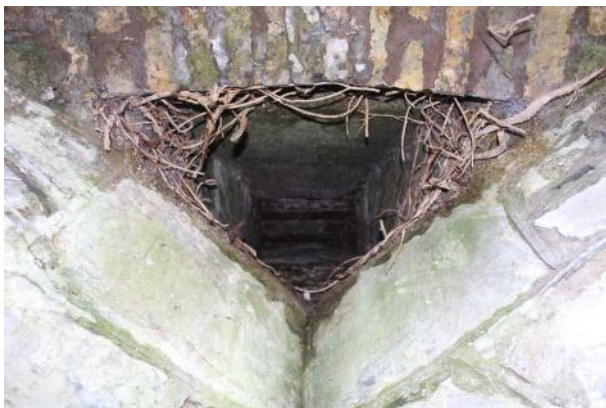
View up into arch from outside, showing squinch hole.
