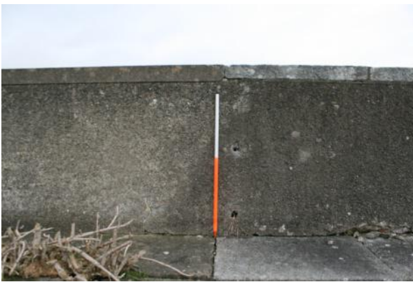
Detail of joint between old and rebuilt segments of parapet wall.
