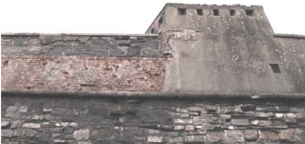
Area A, external view of SE cavalier looking SW
