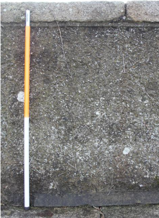
Detail of parapet wall.
