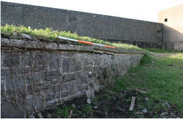
W end of the NE-facing rampart retaining wall.
