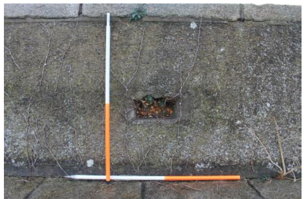
Detail of rectangular niche in parapet wall.
