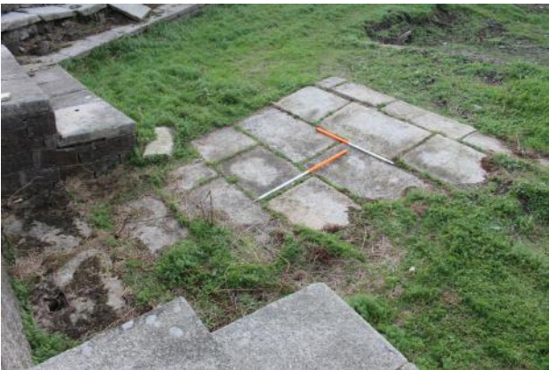
Gun emplacement platform.
