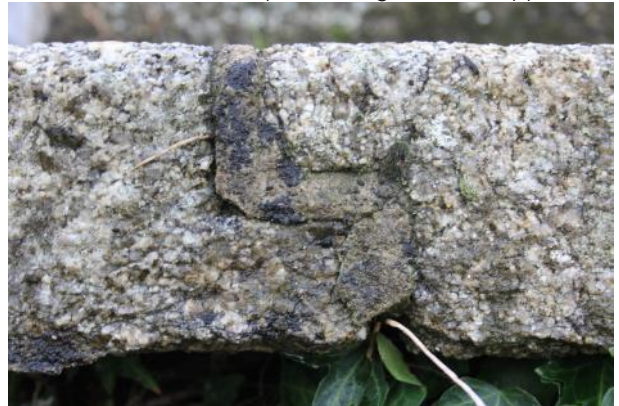
Details of joggle joint with strap pointing on granite walkway slab.
