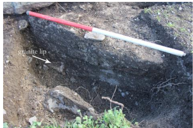
W face of wall. Note granite lip and thick mortar layer on face of wall.
