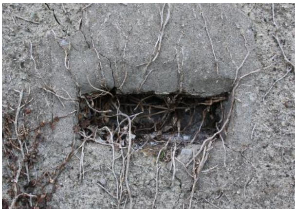
Detail of rectangular niche in SW wall.
