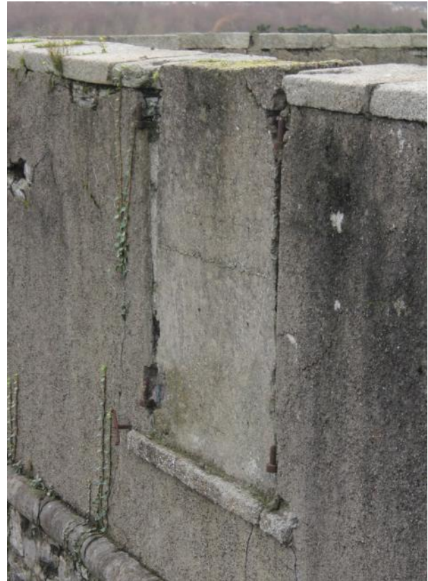
External view of gun embrasure in E wall of SW bastion. Note metal hinges at base of gun embrasure.
