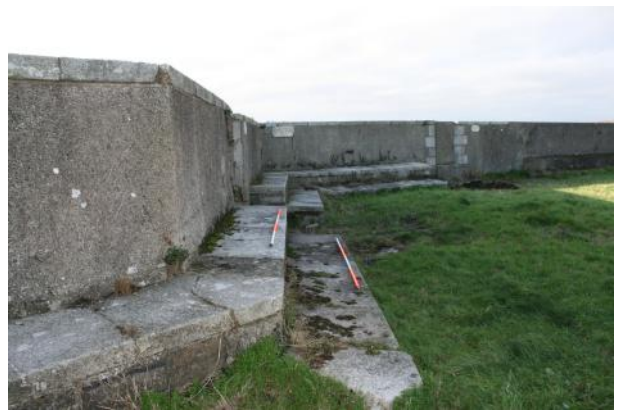
General view of stepped walkway in NW bastion. Looking W.
