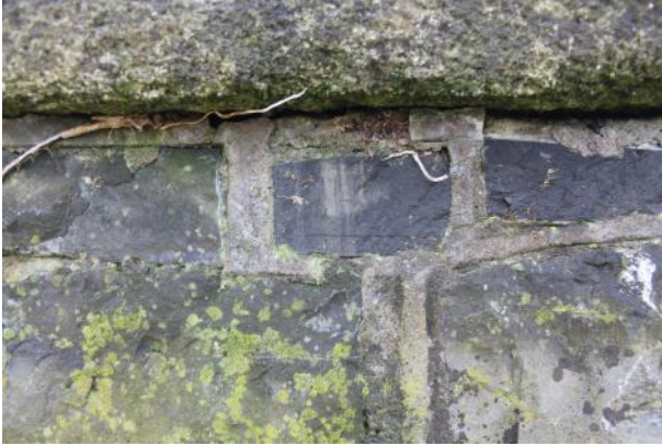
Detail of cement strap pointing on retaining rampart wall.
