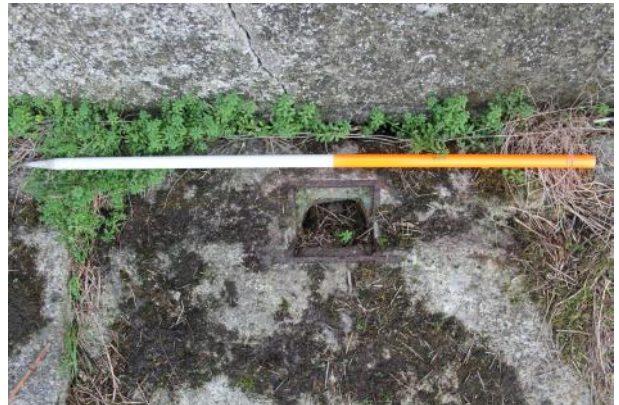
Detail of drain in E end of gun emplacement platform.
