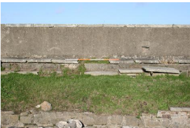
Detail of granite slab steps at E end of S-facing rampart.
