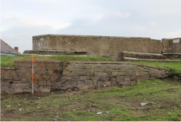
W-facing segment of the rampart retaining wall.
