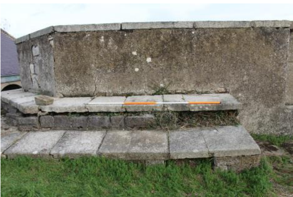
Rampart walkway to N of gun emplacement.
