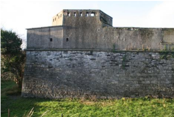
Area A, external view of SE cavalier looking N
