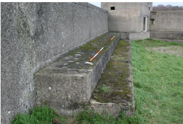
Detail of concrete section of walkway running SE of cavalier.
