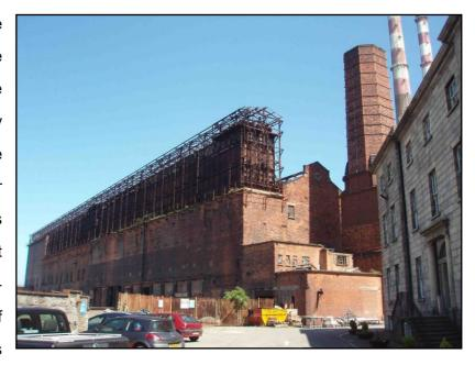
ominous cracks are visible at the northern end of the structure. It is in terrible condition and urgently requires a full survey and restoration. The plant is a Protected Structure, but not a Recorded Monument, and also appears on the Dublin City Industrial Heritage Record 2007.
