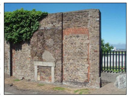
elements above, with two very large windows situated to either side overlooking the harbour. Timber lintels and brick surrounds are still visible, although these features were all filled in, probably during the construction of the military fort in 1778 or soon after.
