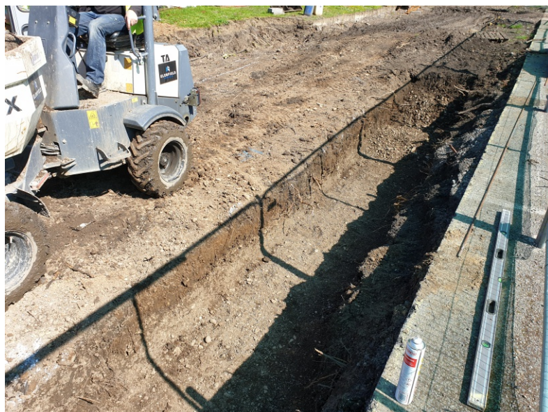
Service trench to west of site
