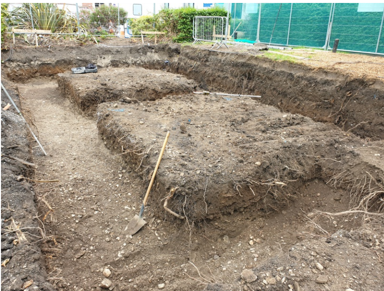
Foundations for new services block
