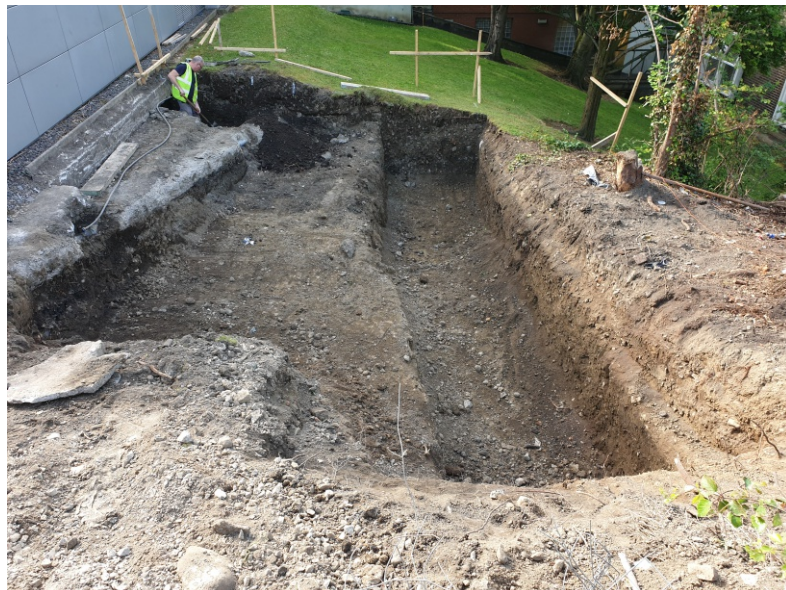
Foundations for extension to old services block
