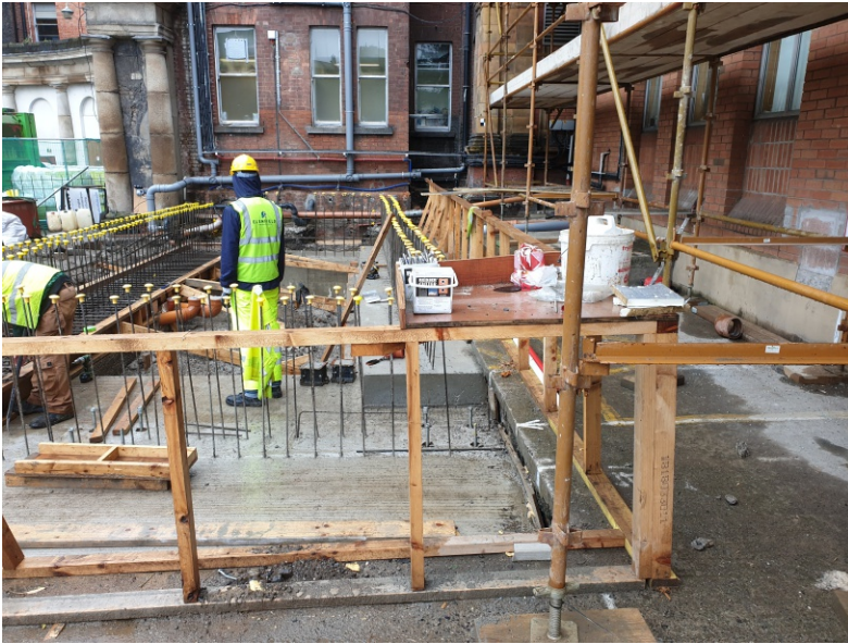
Construction of foundation for new clinical extension
