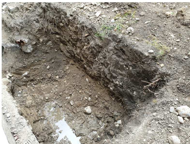
Service trench to east of site
