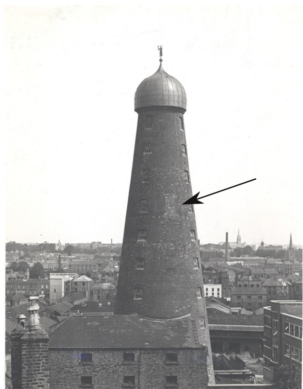
Photograph of tower with external buildings from mid-20th century (Guinness Archives ref GDB.EN02.0001.02 mas). Arrow points to infilled doorway to earlier platform.
