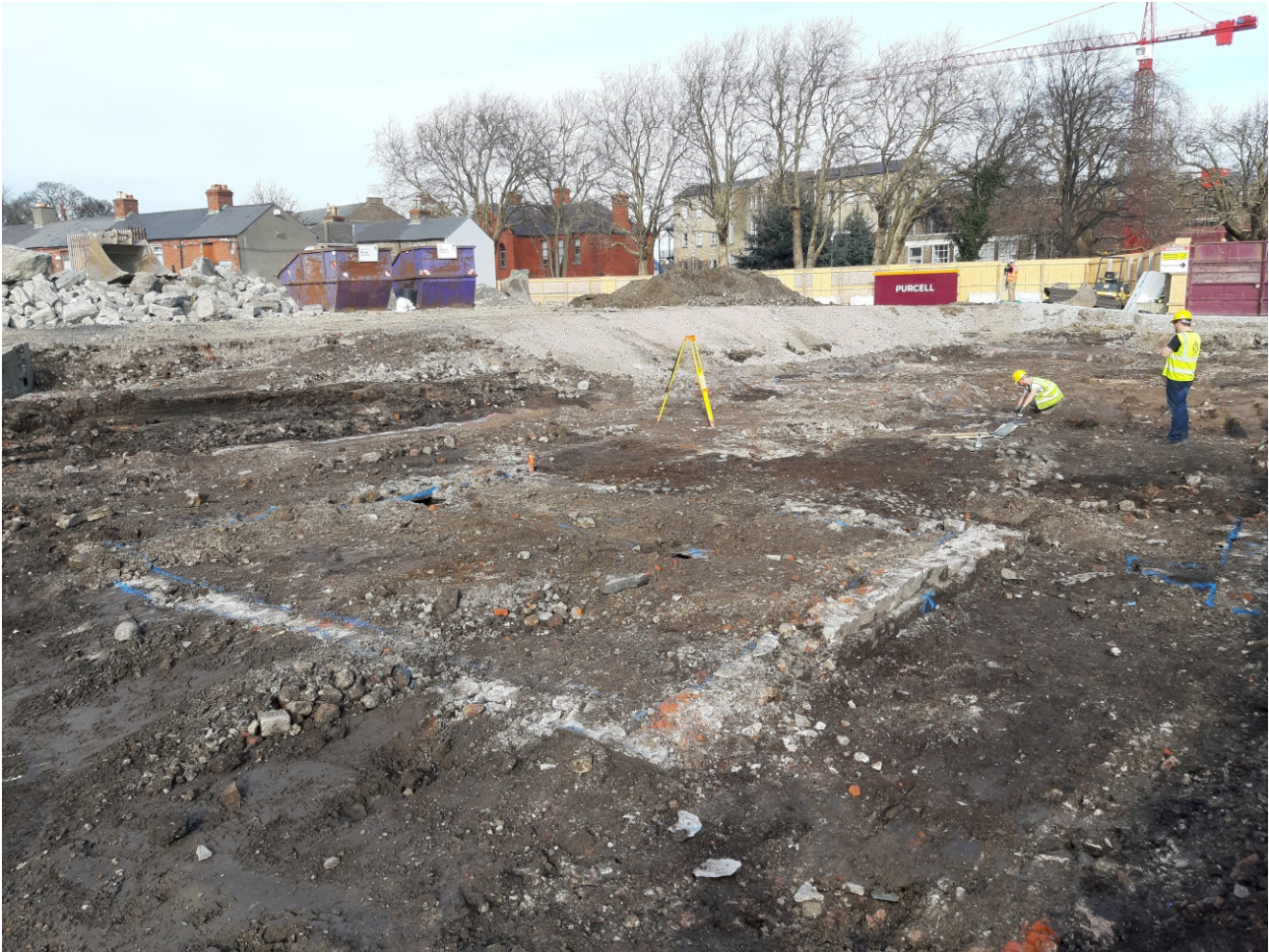
Wall foundations of the 18th century building
