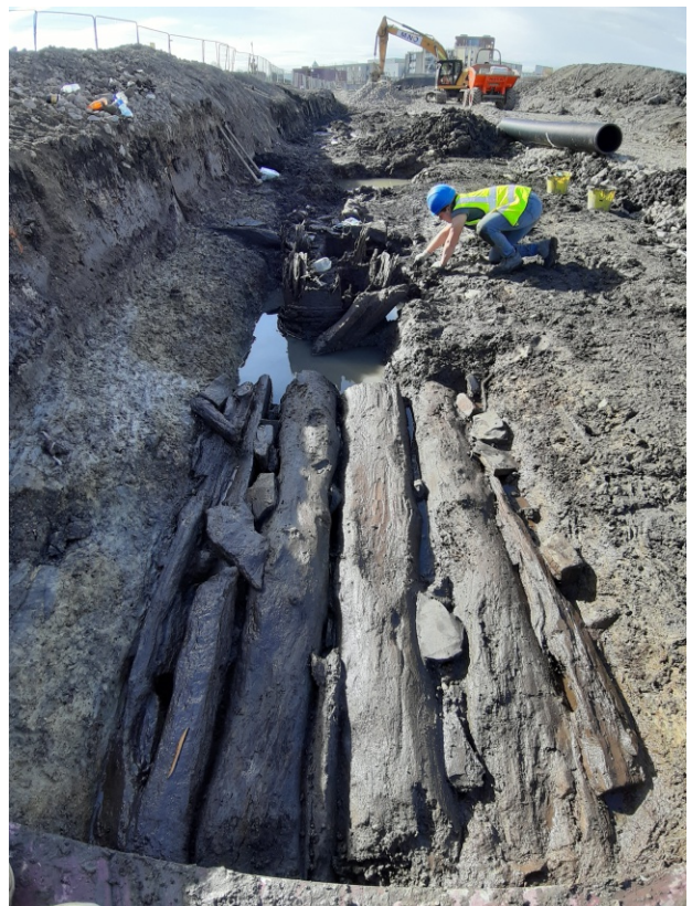
Above, Phase 2 pump or hydraulic ram: Mid ex. Facing South. Both barrels and pipe (F008). Fills: F003 to the east & F004 to the west. Below, excavating the phase 2 pump
