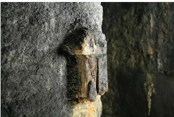
cellar 1 lock mechanism at doorway
