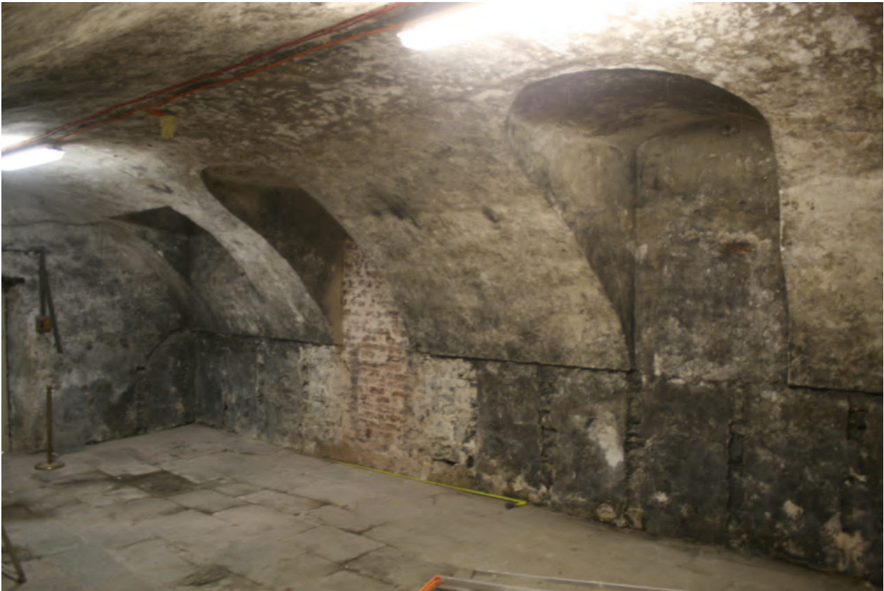
Works area and surrounding room and openings, following removal of plaster
