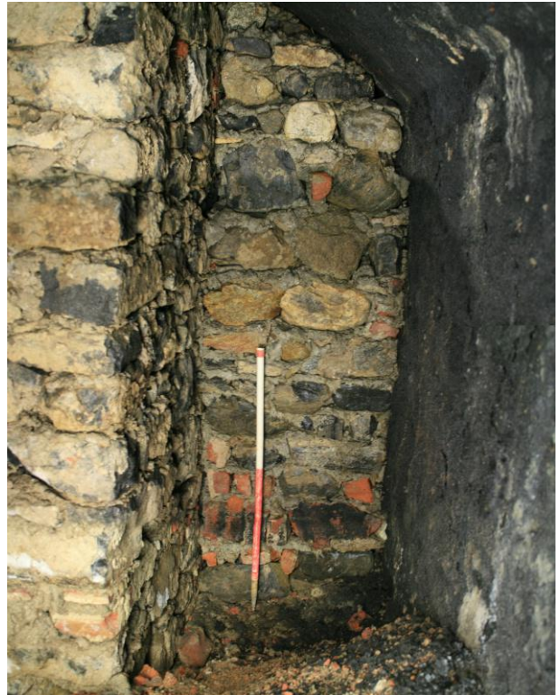
cellar 1 wall 7 facing north. Note how cellar wall to right of image is blackened with coal dust, while wall 7 and wall 5 (to left of image) is not, indicating the coal cellar became disused following construction of wall 5
