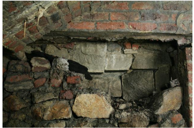
cellar 2 north facing, showing original entrance to cellar
