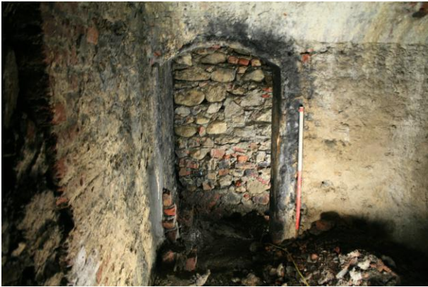
cellar 2 east facing, showing door to cellar 1
