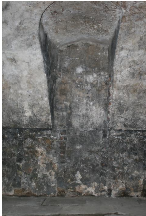
Works area prior to any intervention, showing plaster
