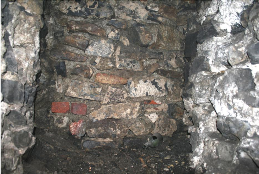
View straight through hole, showing original 16th century broken masonry to left and right, and brick and stone wall blocking far end of passage to rear
