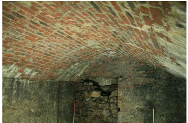
cellar 2 north facing, showing roof
