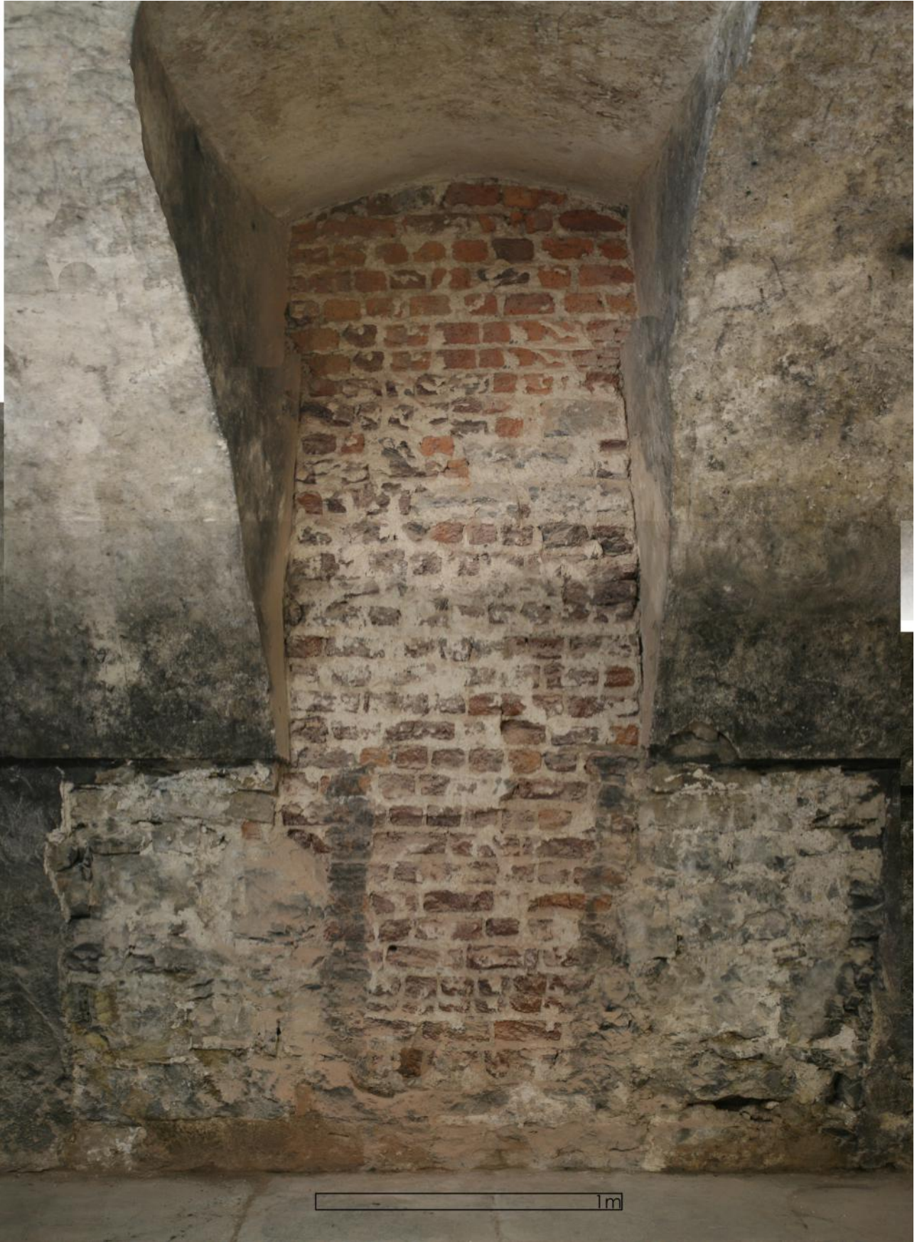
Rectified photograph (ie. to scale) of works area following removal of plaster, showing cut in 16th century wall
