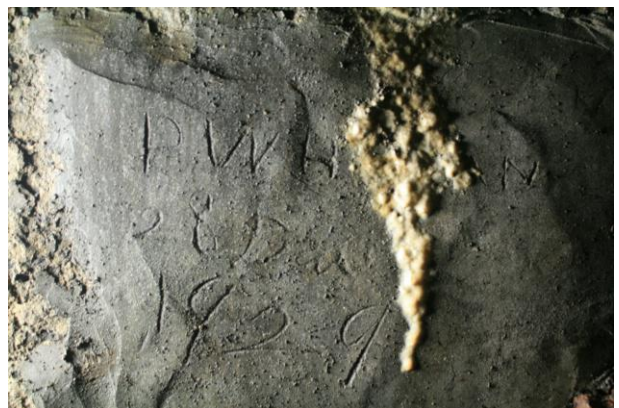
cellar 2 north facing, showing graffiti detail
