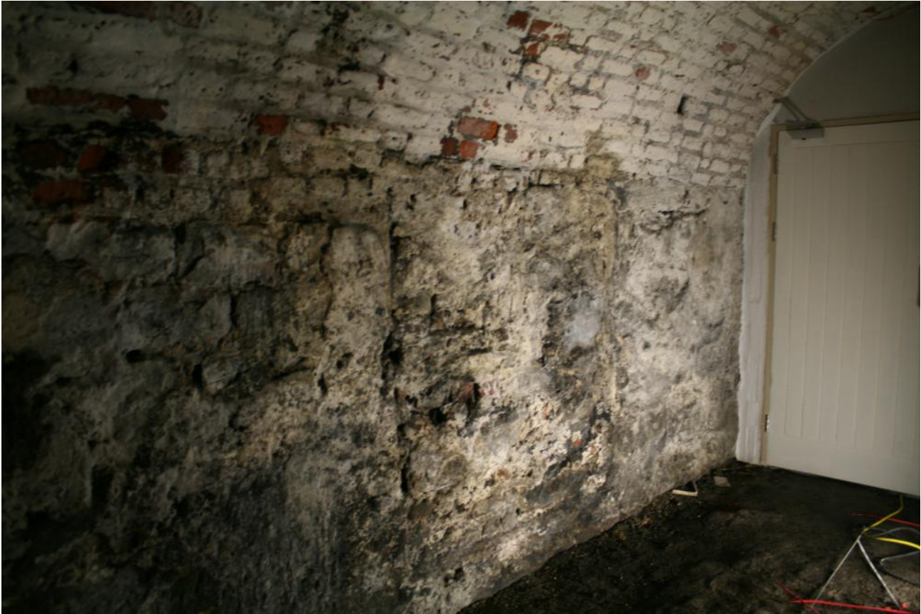
northwestern flanker basement wall, showing blocked 16th century doorway
