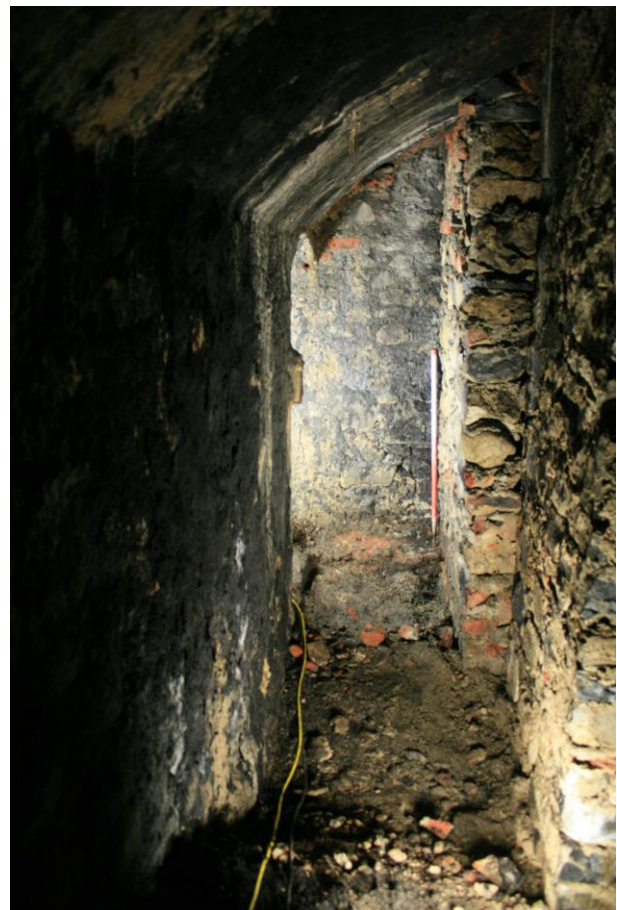
View northwards into cellar 1
