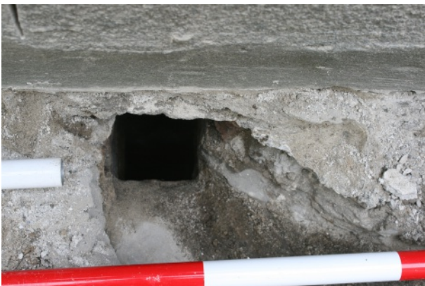
Detail of portico drain outlet below parapet
