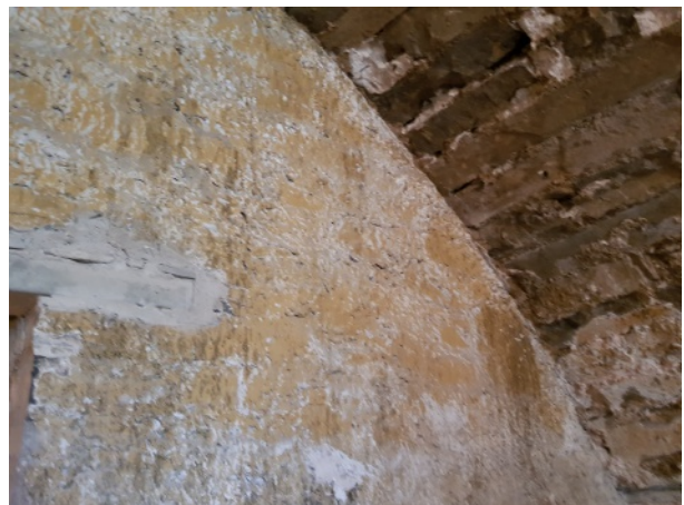
Plaster type F: ochre paint finish of 20 th century date on the west wall of Room B7
