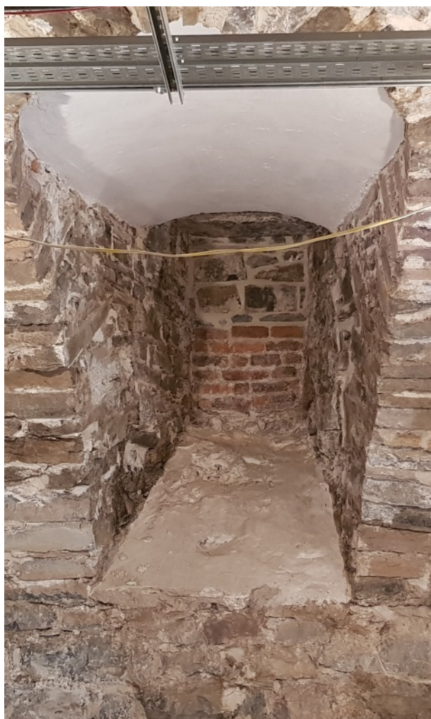
Blocked window of Room B7, following conservation
