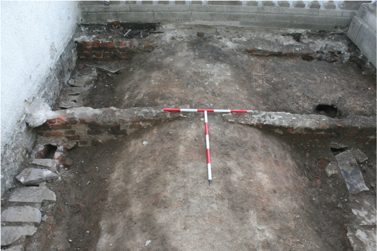
Excavation of portico showing brick crown of coal cellar vault, brick walls constructed over cellar vault, and drains
