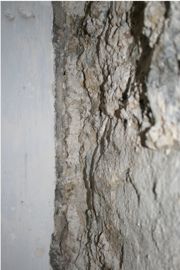
Close-up of late 16th century harling (plaster type E) in B6 plaster over an uneven subsurface, such as that
