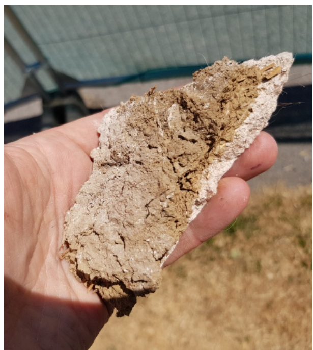
Close-up of earth showing twigs and straw
