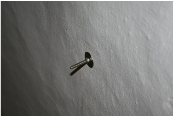
4mm stainless steel restraint fixing into clay/loam plaster
