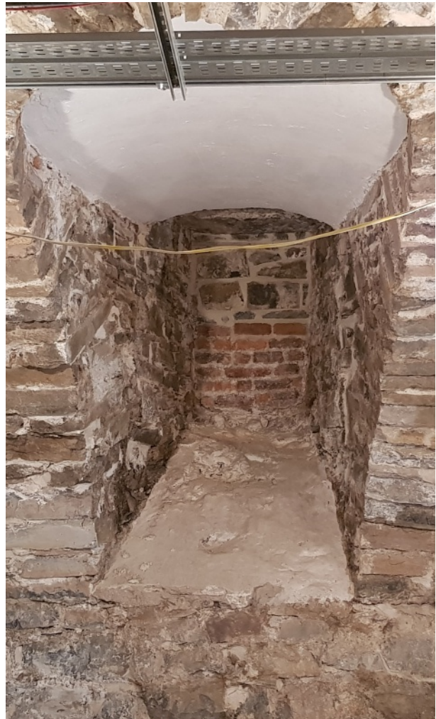
Type B lime plaster, or early 18 th century date, identified at base of window embrasure in B7 (above) and directly above wooden lintel in doorway of B10 (below)
