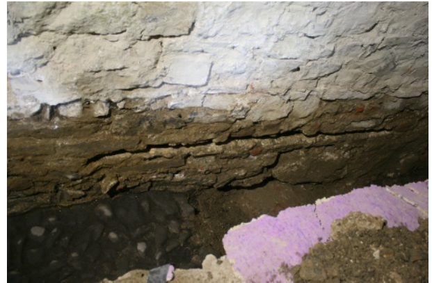
Excavation pit 3 showing slot in dividing wall
