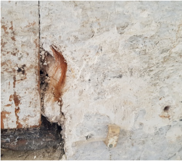
Plaster type D, late 18th century plaster, in Room B6, showing reddish hair inclusions
