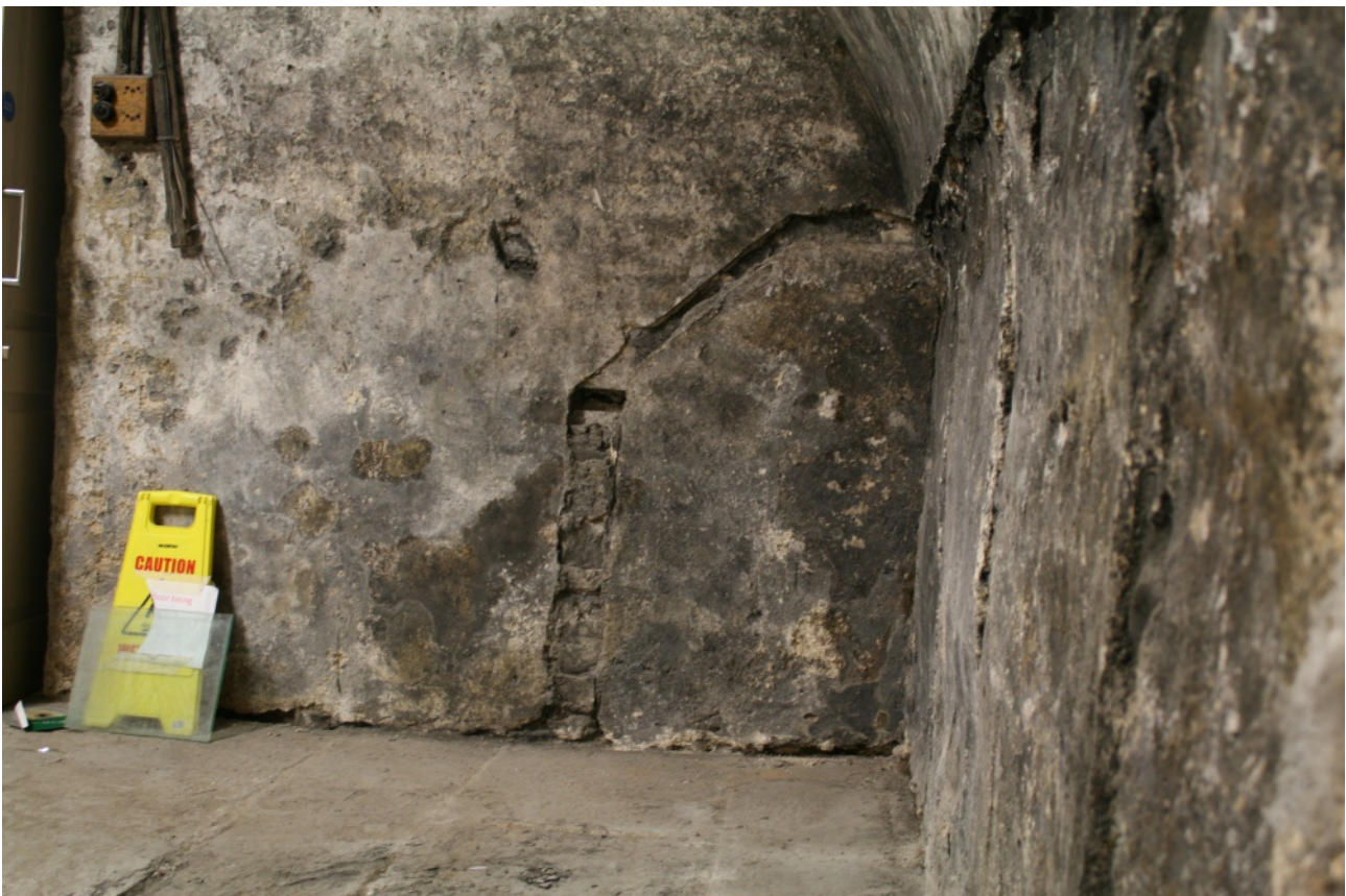
Plaster type C, 18th century lime and aggregate plaster, in Room B8. The plaster is later than the former coal bunkers, whose outlines can be identified in the walls
