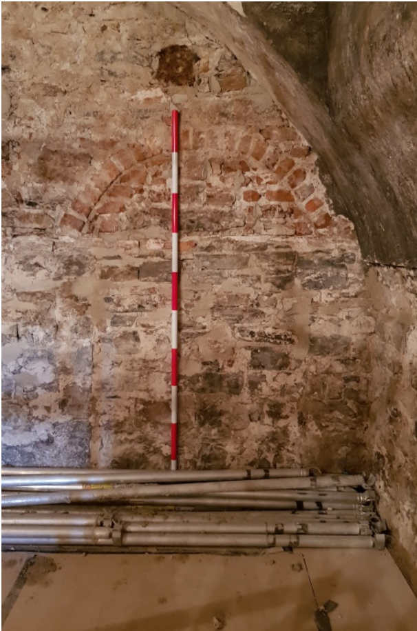
Blocked doorway in western wall of Room B8
