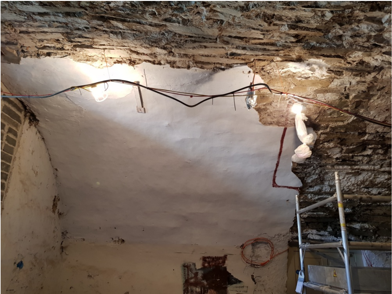
The largest surviving section of the earth mortar plaster, in situ on the north wall of B7
