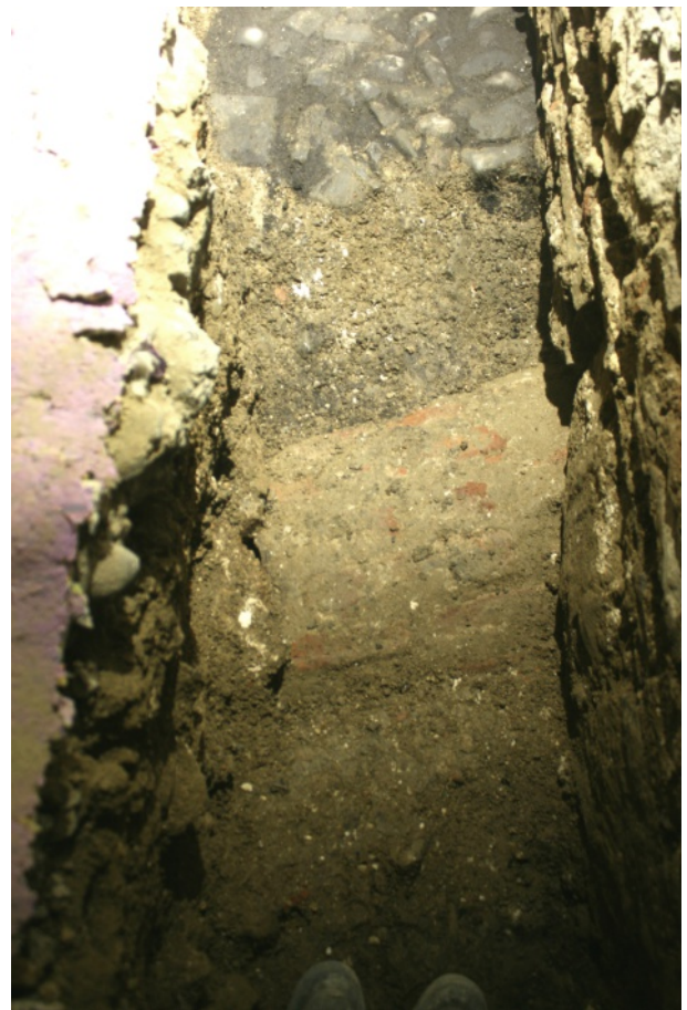
Excavation pit 3 showing brick crown of drain culvert cut through cobbled floor
