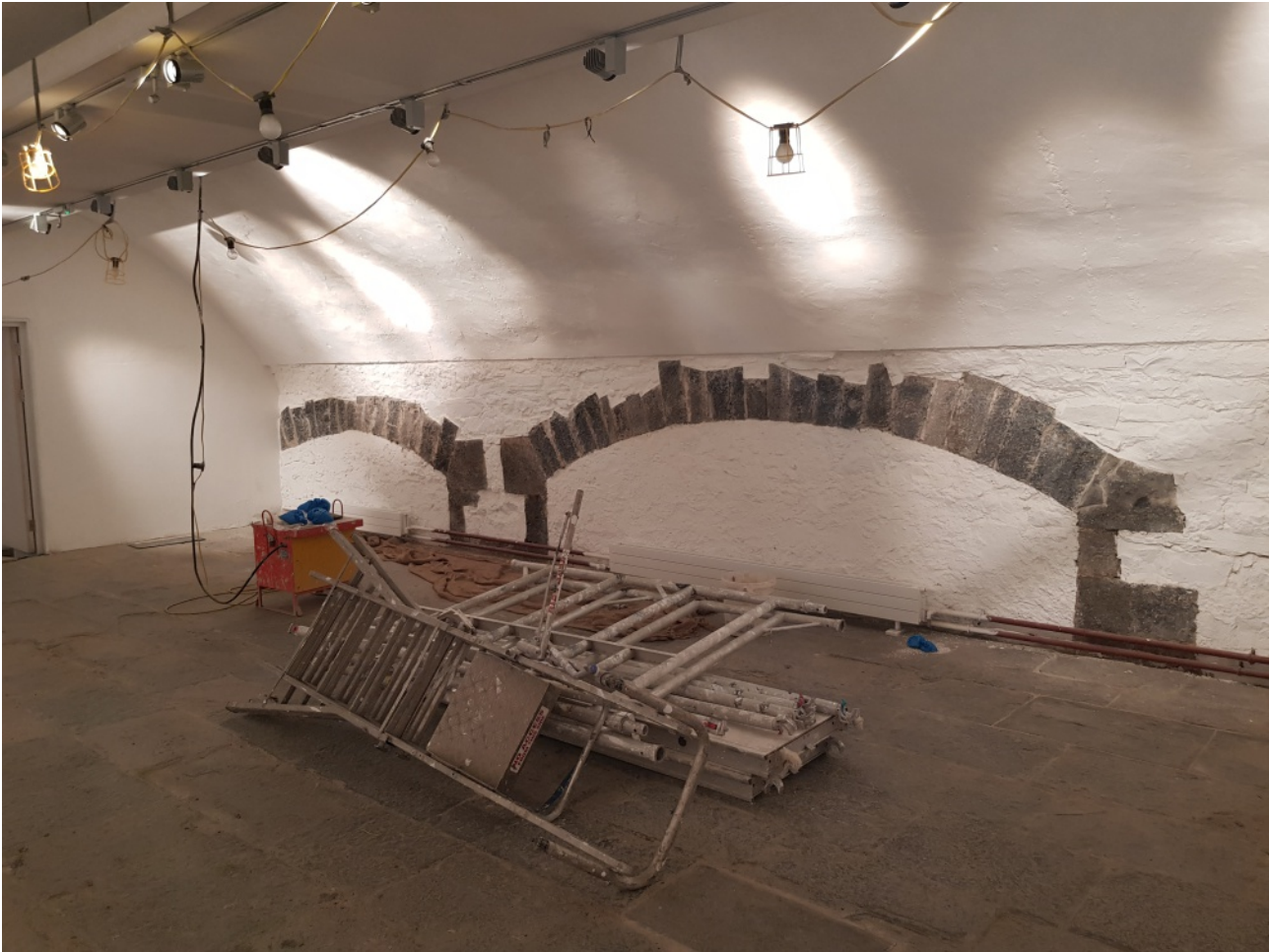
Fireplace arches in Room B8 south wall following conservation
