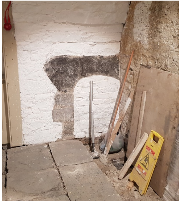
Bake oven, following restoration works
