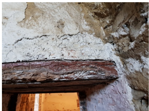
Type B lime plaster, or early 18 th century date, identified at base of window embrasure in B7 (above) and directly above wooden lintel in doorway of B10 (below)
