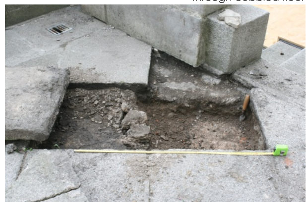
Excavation of portico showing layers below paving stones
