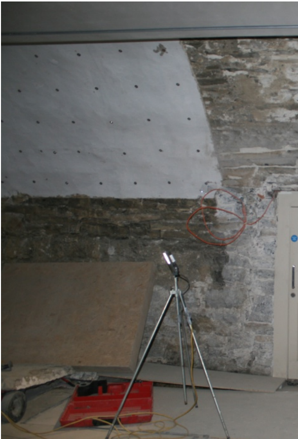
Conservation of clay/loam plaster in room B7
