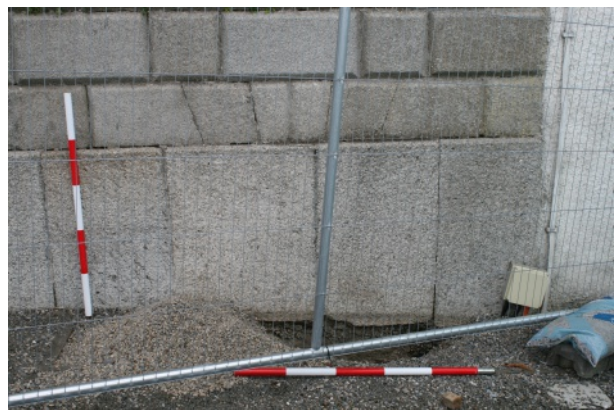
Voussoirs at entrance to former coal cellar
