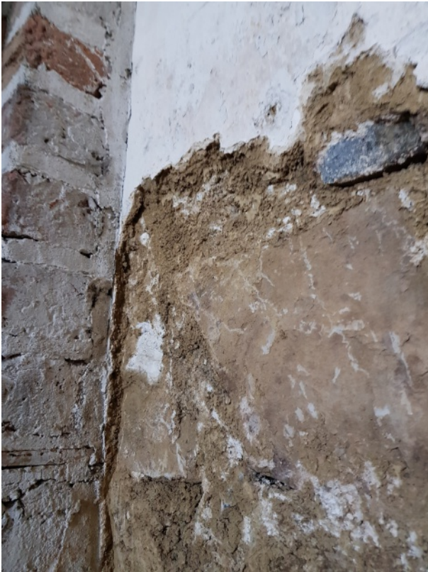
Earth mortar plaster in situ on south wall of B10
