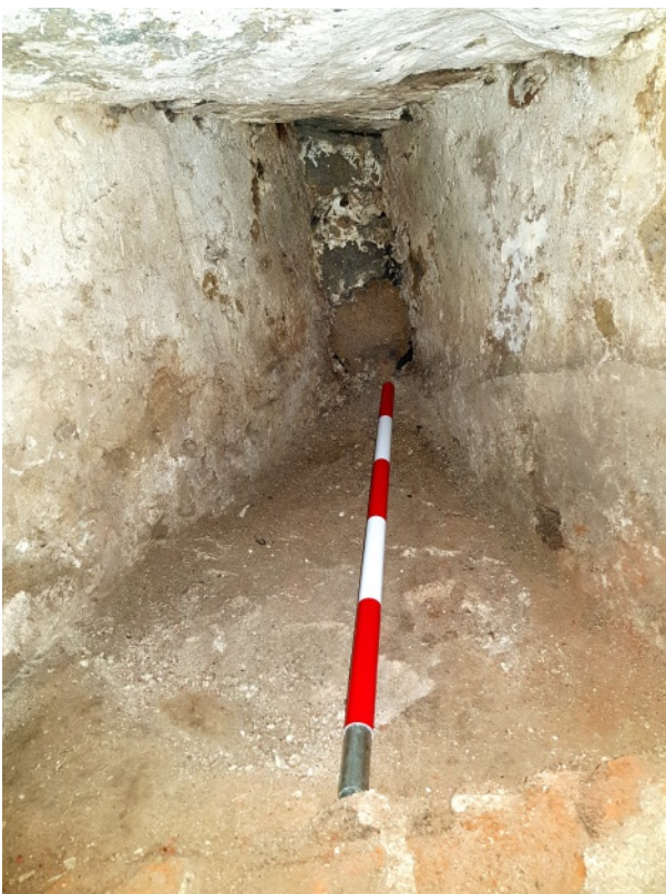
Northern gunloop in tower B10, showing circular gunloop filled with clay in the back of the loop
