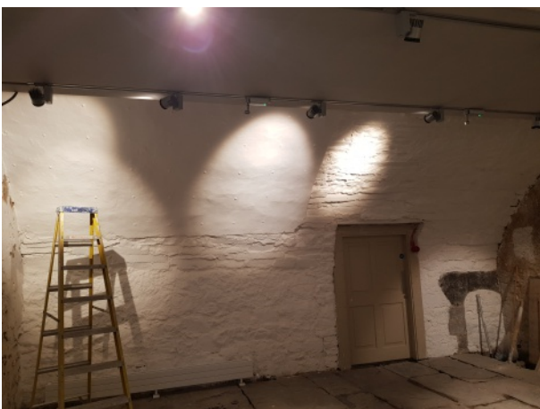
Conserved clay/loam plaster in room B7
