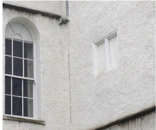
Above, on the left 18th century sash window; on the right sealed 16th century mullioned window
