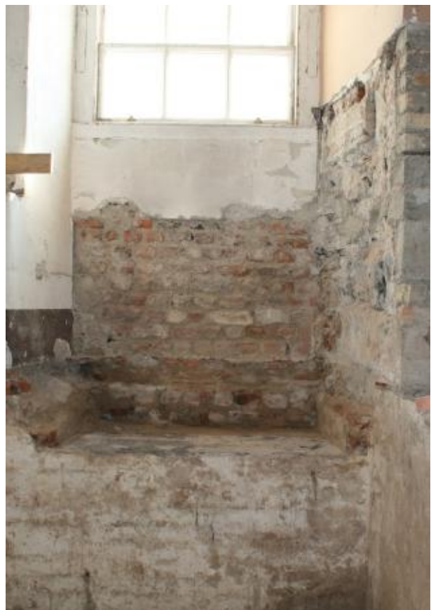
Above: decorative niche or cabinet, showing partially-replastered cavities to hold shelves. Facing southwest Below: 18 th century window showing earlier phase with limestone sill in lower part of image, facing east
