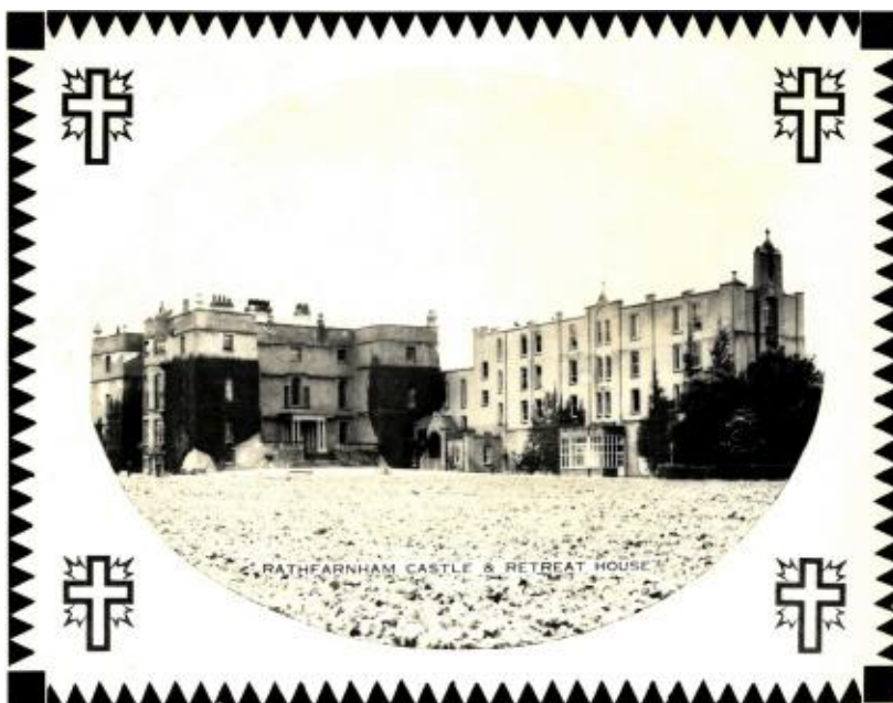
Above and left: 20th century photographs showing the great wing constructed by the Jesuits. Above: north-facing view of construction of southern junior wing 1925. Left: southwest facing view of front of the castle and the northern wing 1940. South Dublin County Council
