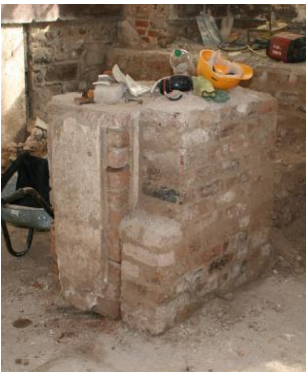
Above: northernmost structural support for ceiling, facing north. It is abutted to the left by a later floor support Below: second from north structural support (2) for ceiling, facing northeast. It is abutted to the right by a later floor support
