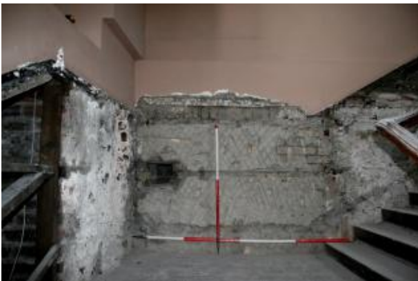
Top: N3 showing arched recess in centre left of image. N4 is visible in the upper right as a cement-blocked opening. N5 is visible as a change of thickness in the wall at the top of the image Middle: N6 showing modern brick blocking a cavity. E8 is visible as a change of thickness of the wall at the top of the image Bottom: N7 showing masonry quoin at bottom of image
