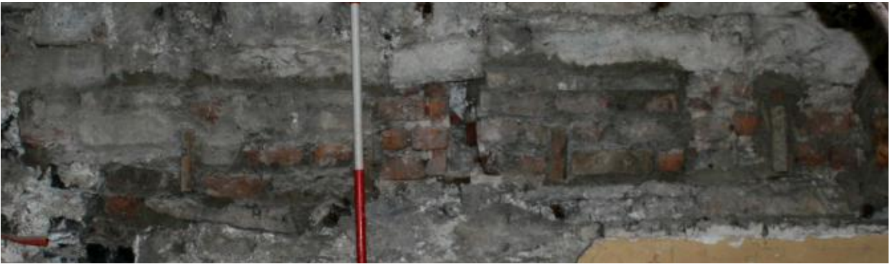
Top: E6 reused timber in gunloop lintel, showing detail of features Middle: E8 showing line of red brick and cavities representing former floor level Bottom right: E8 in west wall showing change in wall thickness at base of window embrasure (W11)
