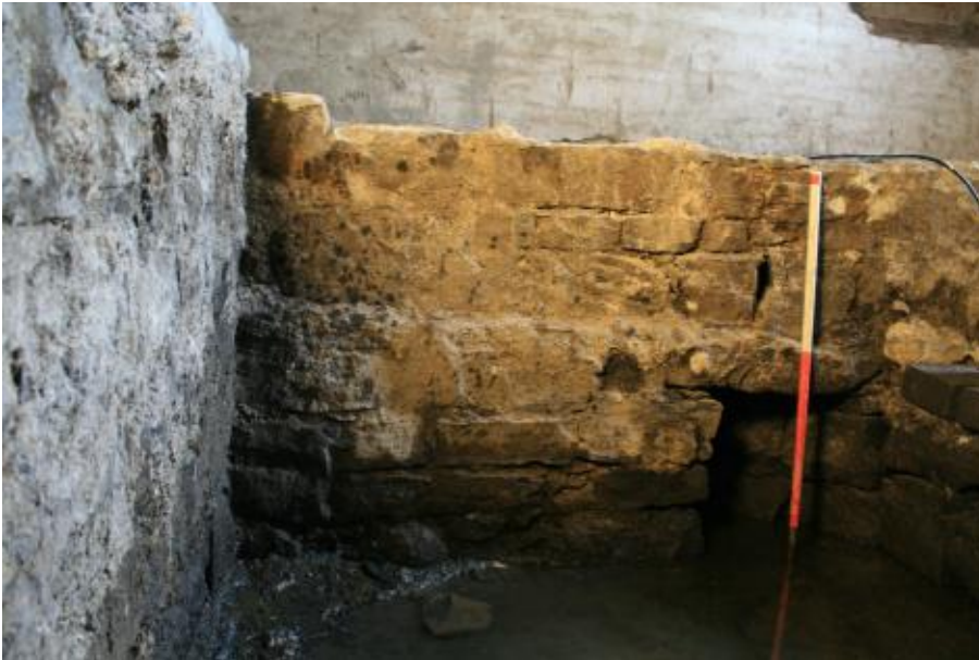
Top left: ledge in the northeast corner of the washpit, facing east. A similar ledge was situated on the opposite side of the washpit, and both ledges may have supported grills or metal shutters at the drain exit and entrance
