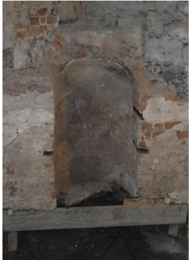
Above: decorative niche or cabinet, showing partially-replastered cavities to hold shelves. Facing southwest Below: 18 th century window showing earlier phase with limestone sill in lower part of image, facing east
