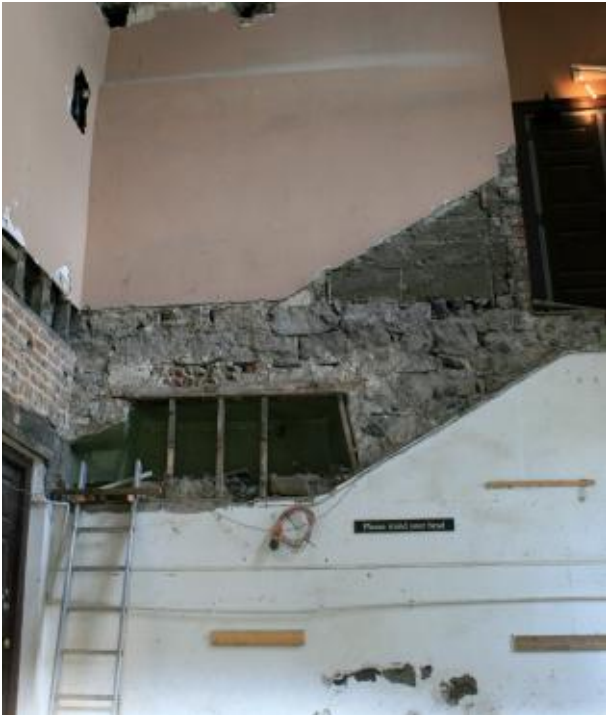
Top: N3 showing arched recess in centre left of image. N4 is visible in the upper right as a cement-blocked opening. N5 is visible as a change of thickness in the wall at the top of the image Middle: N6 showing modern brick blocking a cavity. E8 is visible as a change of thickness of the wall at the top of the image Bottom: N7 showing masonry quoin at bottom of image
