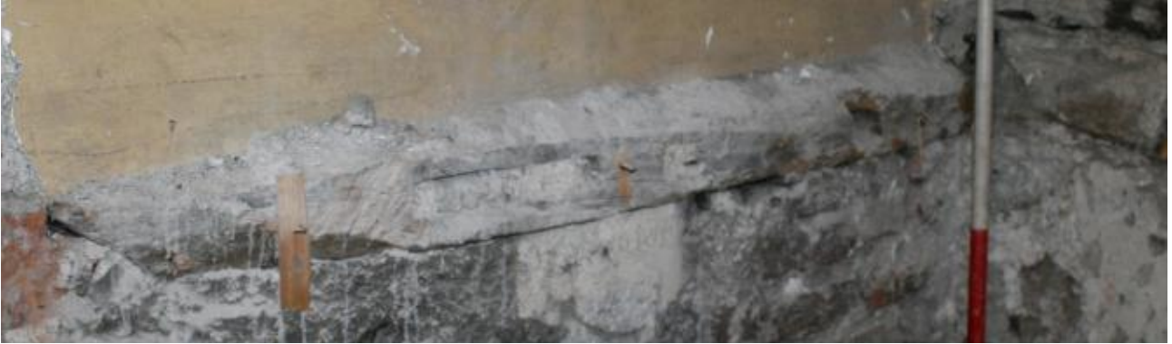
Top: E6 reused timber in gunloop lintel, showing detail of features Middle: E8 showing line of red brick and cavities representing former floor level Bottom right: E8 in west wall showing change in wall thickness at base of window embrasure (W11)
