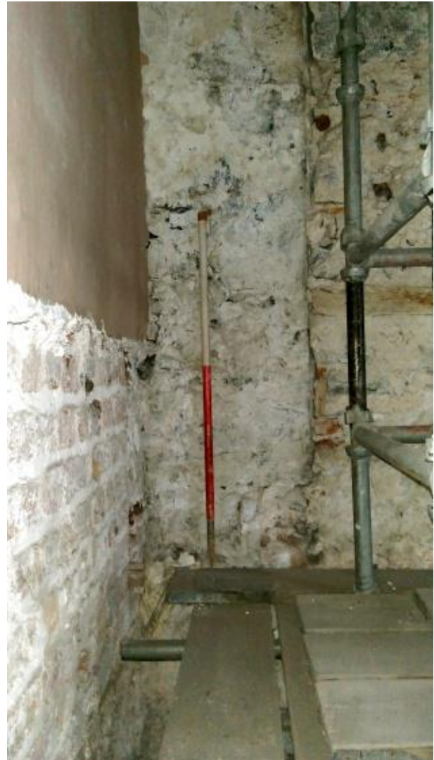
Above: S5, showing upper west jamb stones with brick blocking to right of image Below: S7 18 th century window
