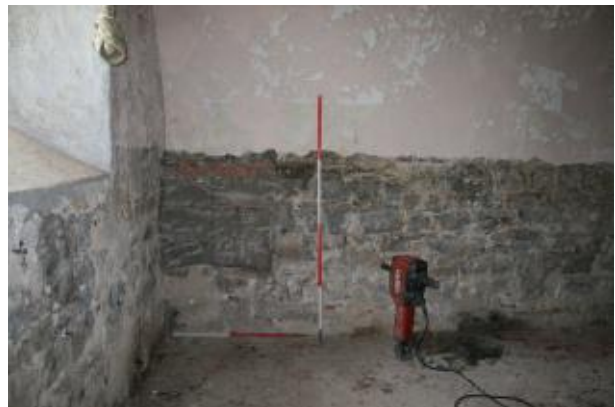
Blocked gunloops in west wall
