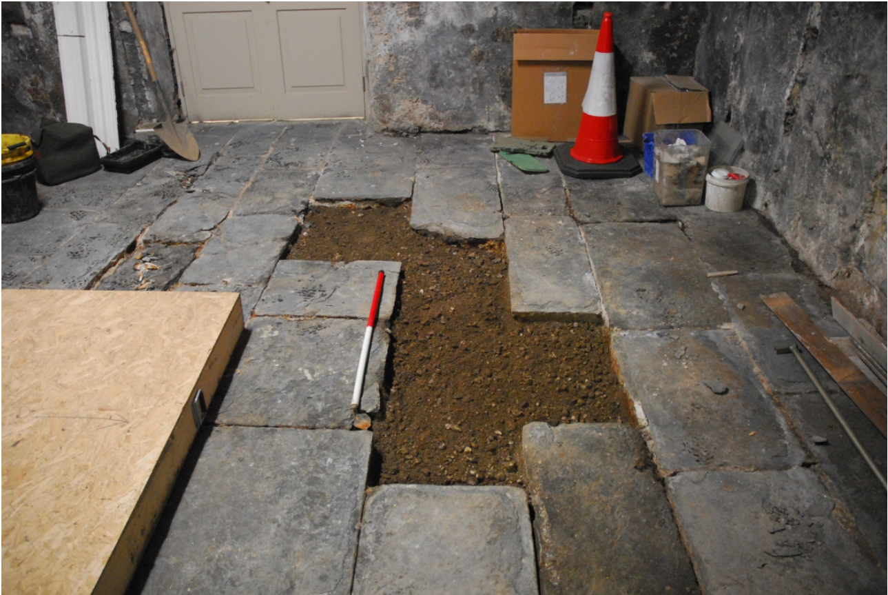
Test-pit 1 prior to excavation, following removal of 18 th century paving stones, facing west
